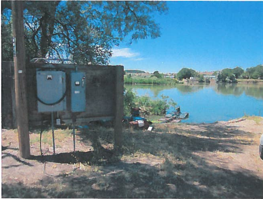
POD looking west. Tag A0018517 on power pole.
