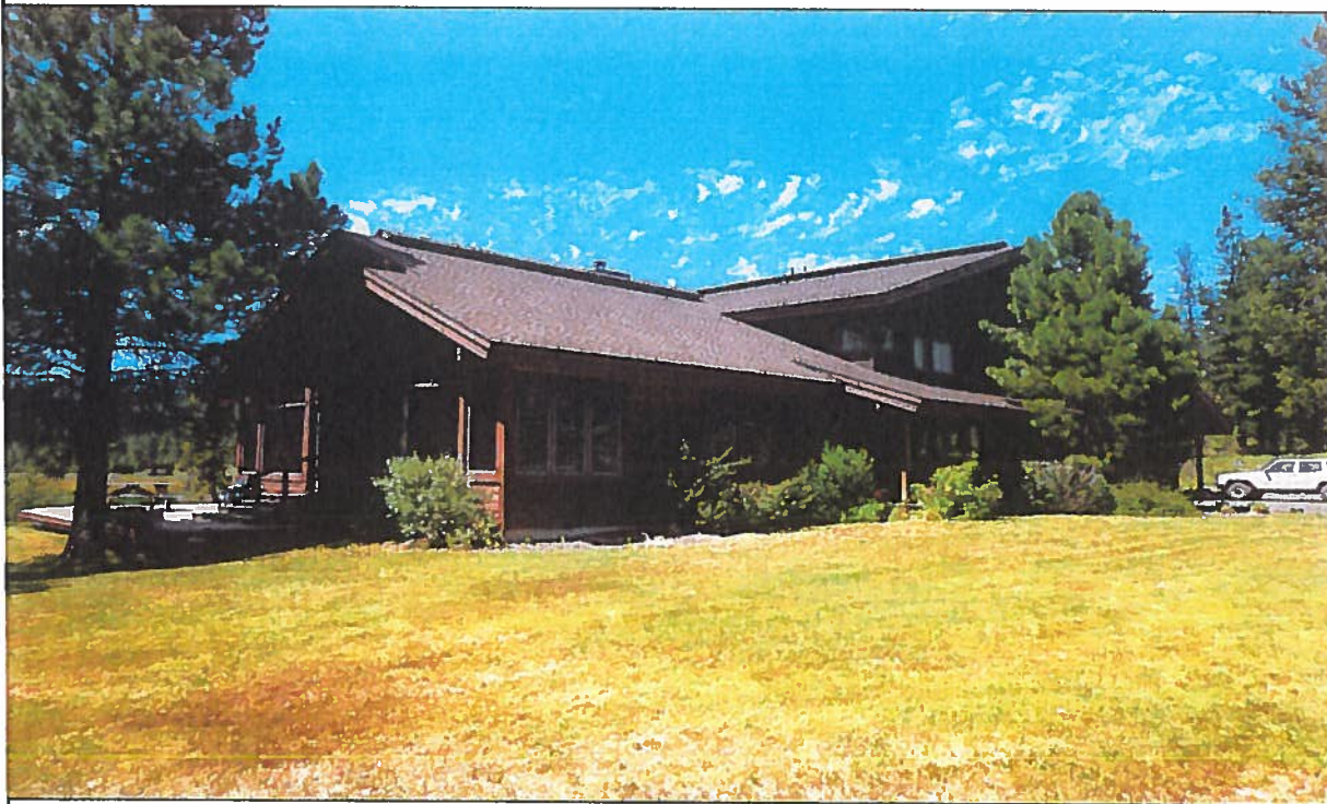
Place of Use: View northwesterly from near the ground water well of the home served by the ground water well.
