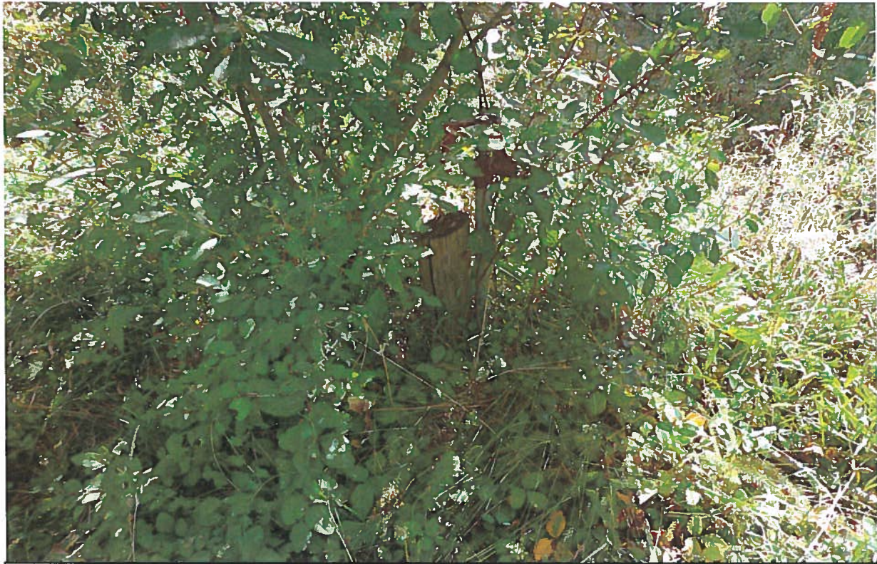
Place of Use: View of the frost-free hydrant near the home.
