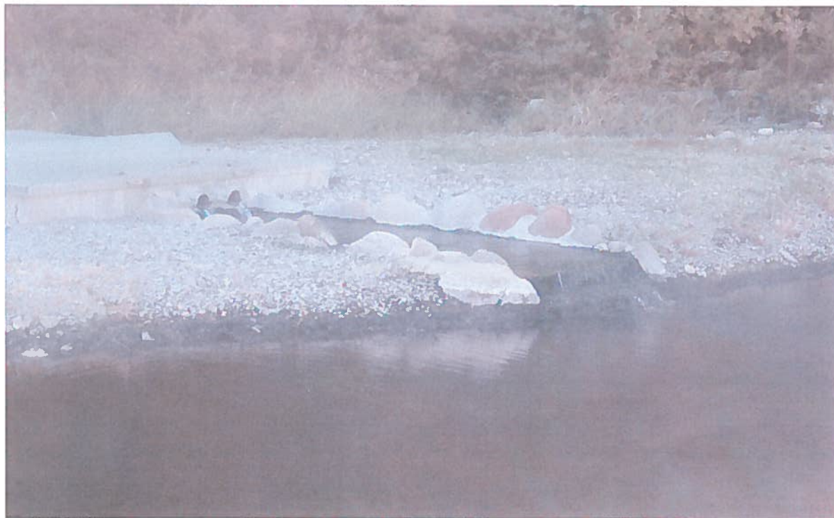
The overflow from spring # 3 into the pond.
