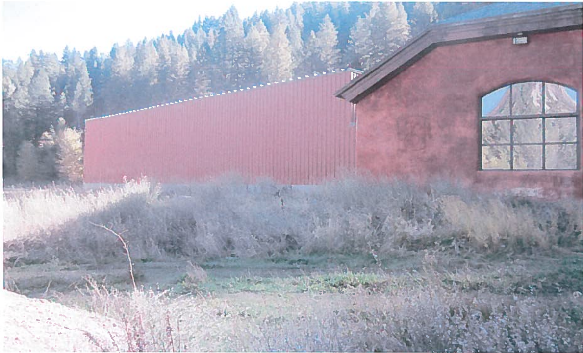
From the area of the overflow pond, looking northeast at the bottling plant, with the attached warehouse in the left.
