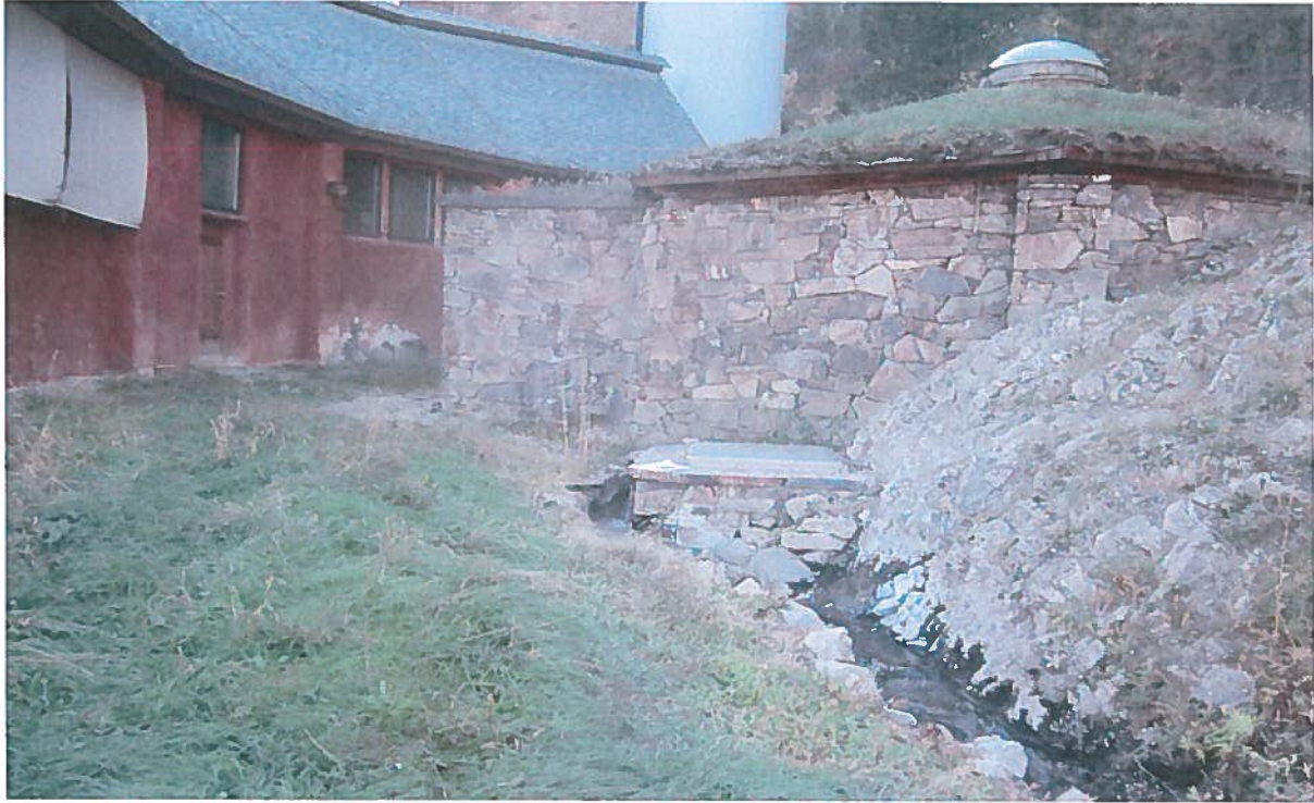
Looking south. The overflow ditch, springs # 1 and 2, and the bottling plant are seen in this view.
