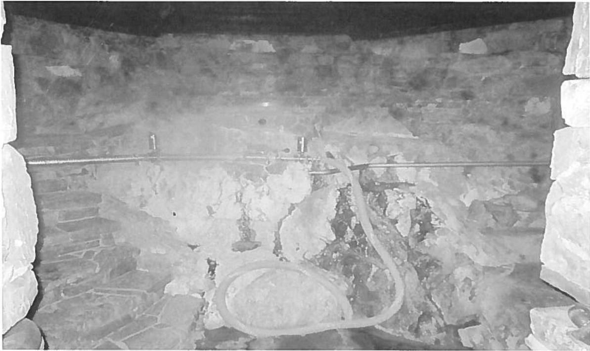
Interior of the main springhouse. Spring is top center.
