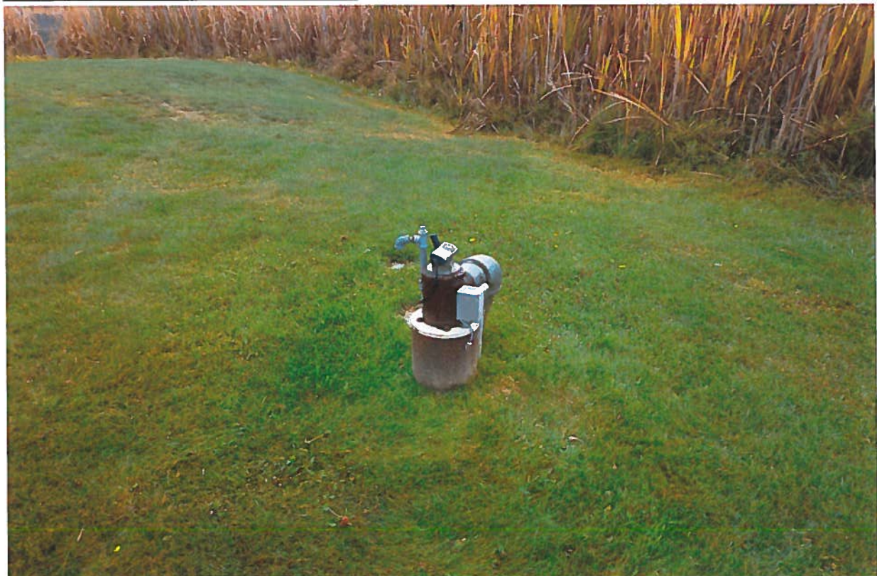
Point of Diversion: View of ground water well adjacent to and north of an irrigation/recreation storage pond located in the 'Cedars 9-Hole Golf Course'.
