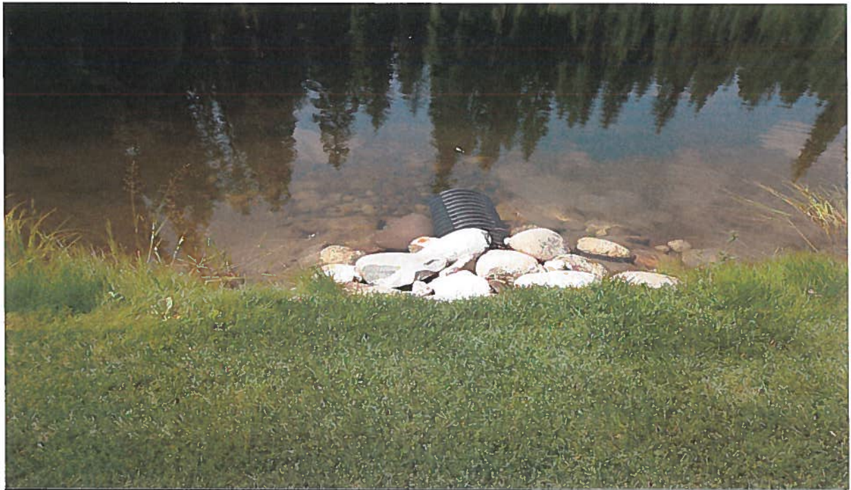
Place of Use: View westerly of the 12" ABS/PVC discharge pipe near the easterly bank of the storage pond.
