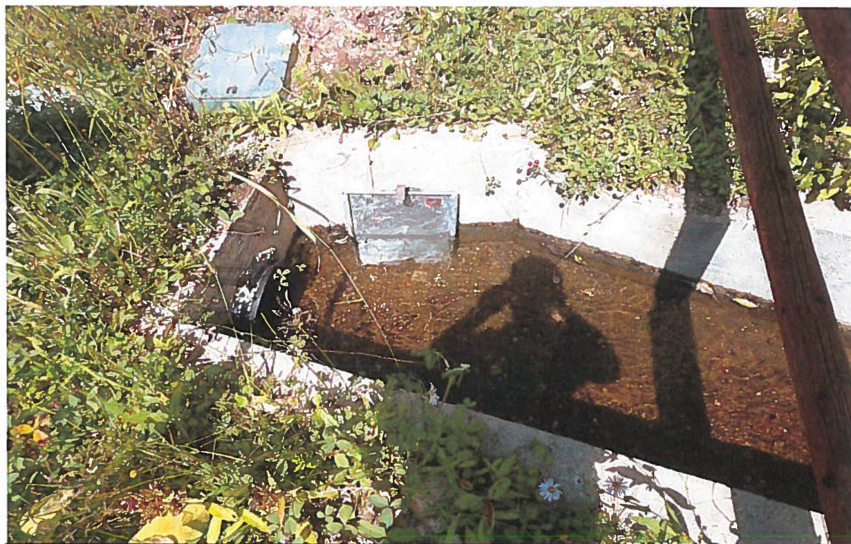
View of concrete collection box between the storage pond and Eastside Road. A 30" CMP culvert pipe across Eastside Road discharges water to the collection box. A section of 12" ABS/PVC pipe discharges water to the storage pond.
