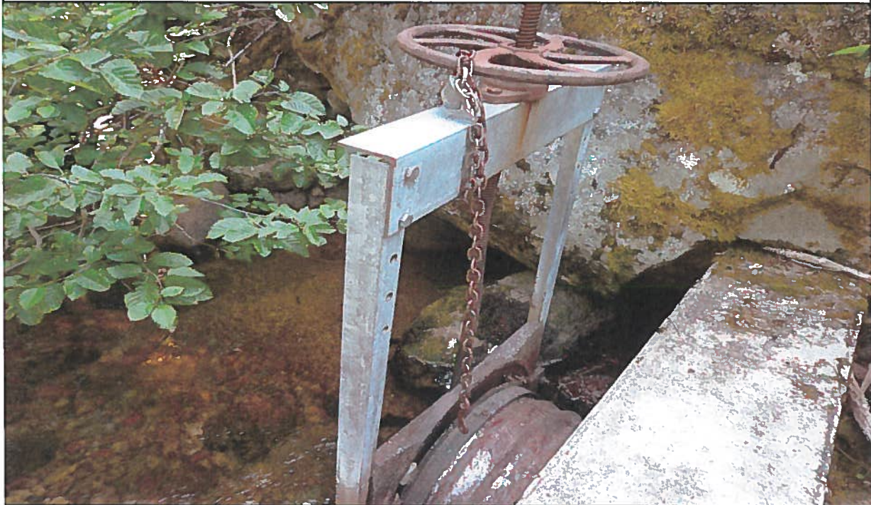
Point of Diversion: View of concrete diversion structure, 36" CMP, and a 36" wheel gate at Fall Creek.
