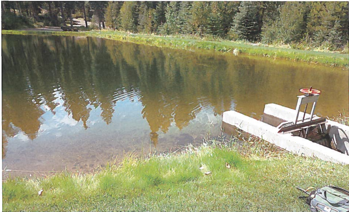
Place of Use: View westerly of the storage pond and the concrete storage pond overflow structure located near the northeasterly corner of the storage pond.
