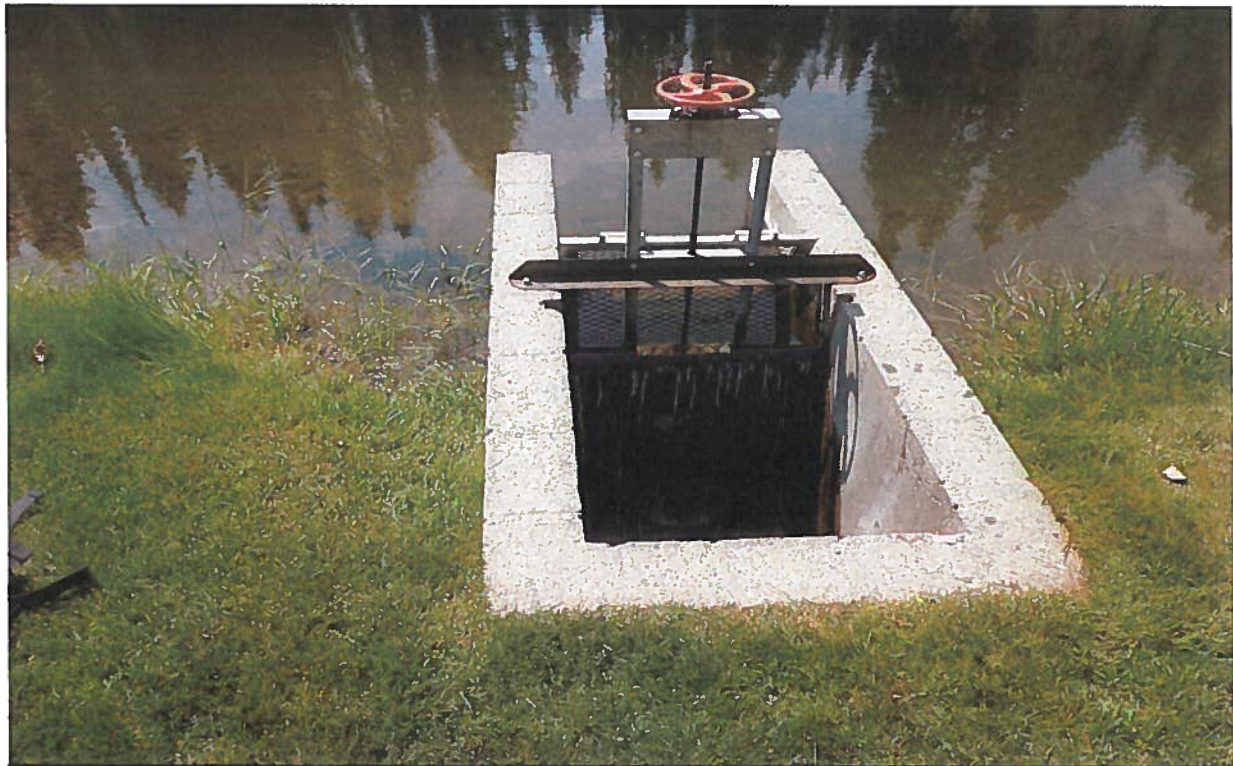
View easterly of the 8' x 3' concrete storage pond overflow structure. Water discharged from the storage pond is conveyed to an open ditch and pipe for discharge back to Fall Creek.
