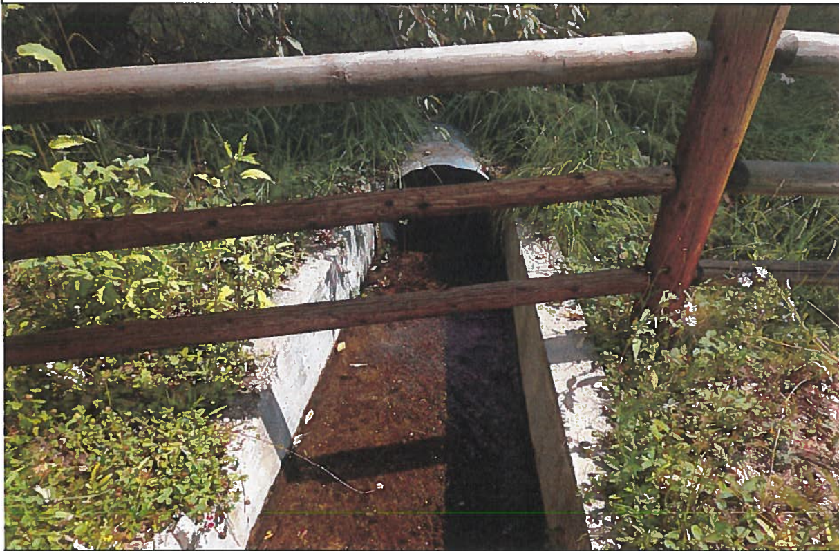
View northerly of a concrete channel and CMP pipe which conveys the storage pond overflow back to Fall Creek.
