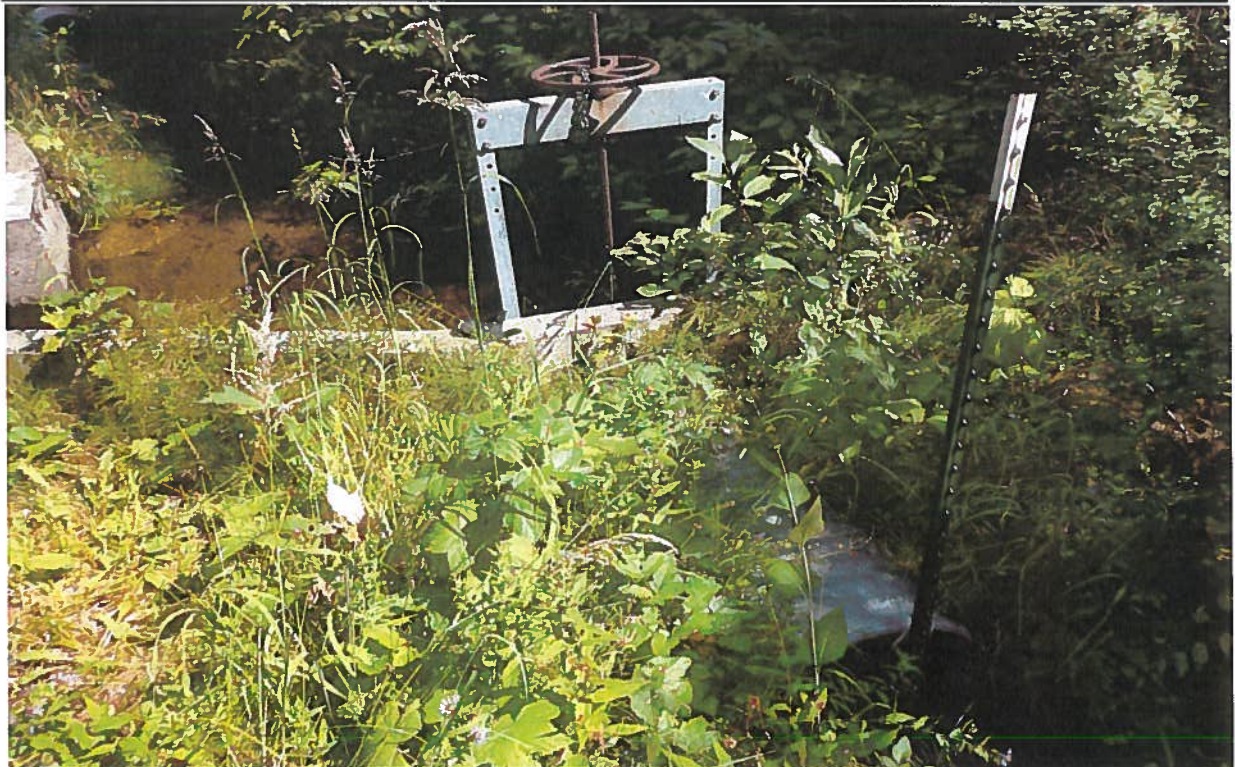
View southeasterly of the concrete diversion structure, 18" CMP, and an 18" wheel gate for the small irrigation ditch.
