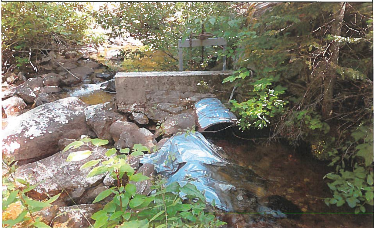
Point of Diversion: View upstream of Fall Creek and the concrete diversion structure.
