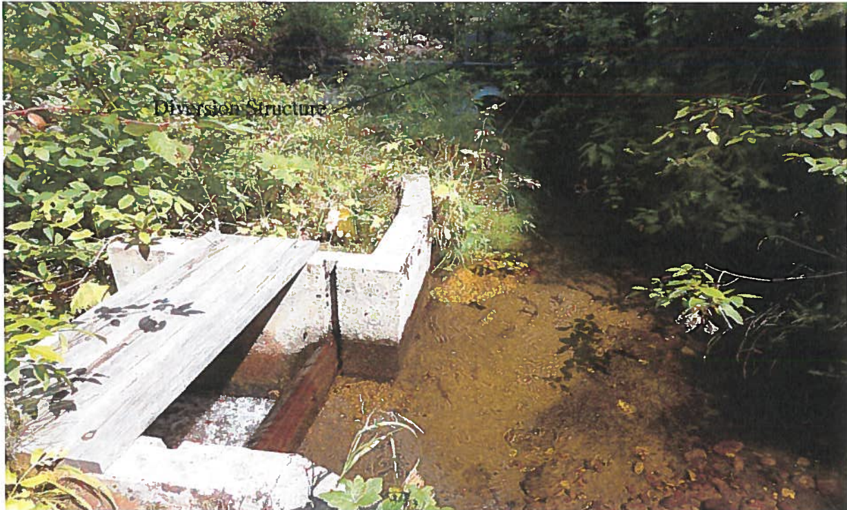
View easterly of the conveyance channel from the Fall Creek diversion. The concrete weir structure is used to maintain static head for the small irrigation ditch used by the right holder and to divert water back to Fall Creek.
