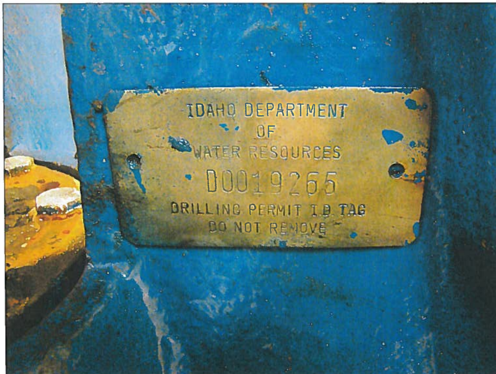
City of Meridian Well #24 IDWR Well ID Tag No. D0019265 located on pump discharge head.
