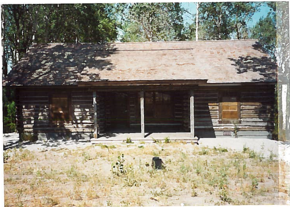
POU cabin Middle bunkhouse
