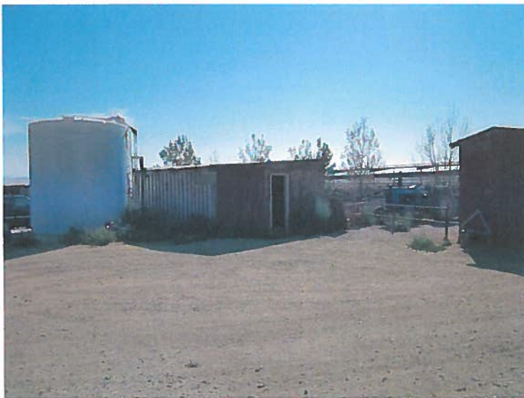
South Well wellhouse
