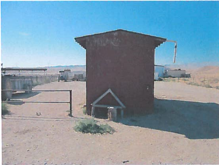
Abandoned well SW of South Well
