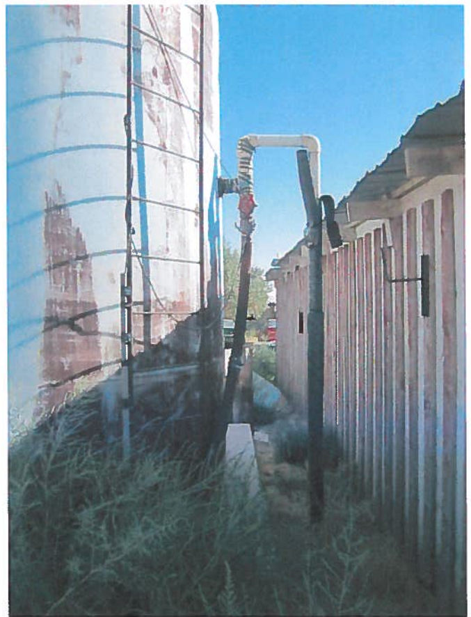
Storage tank and discharge hose
