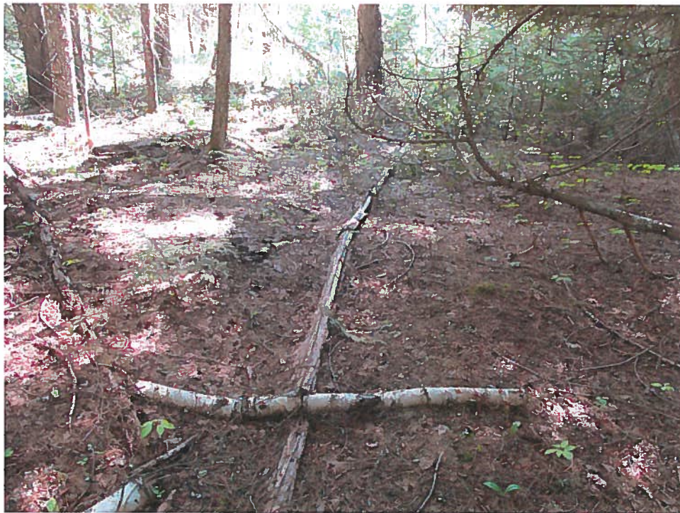
- 1.5 inch PVC line running from the spring to holding tanks
