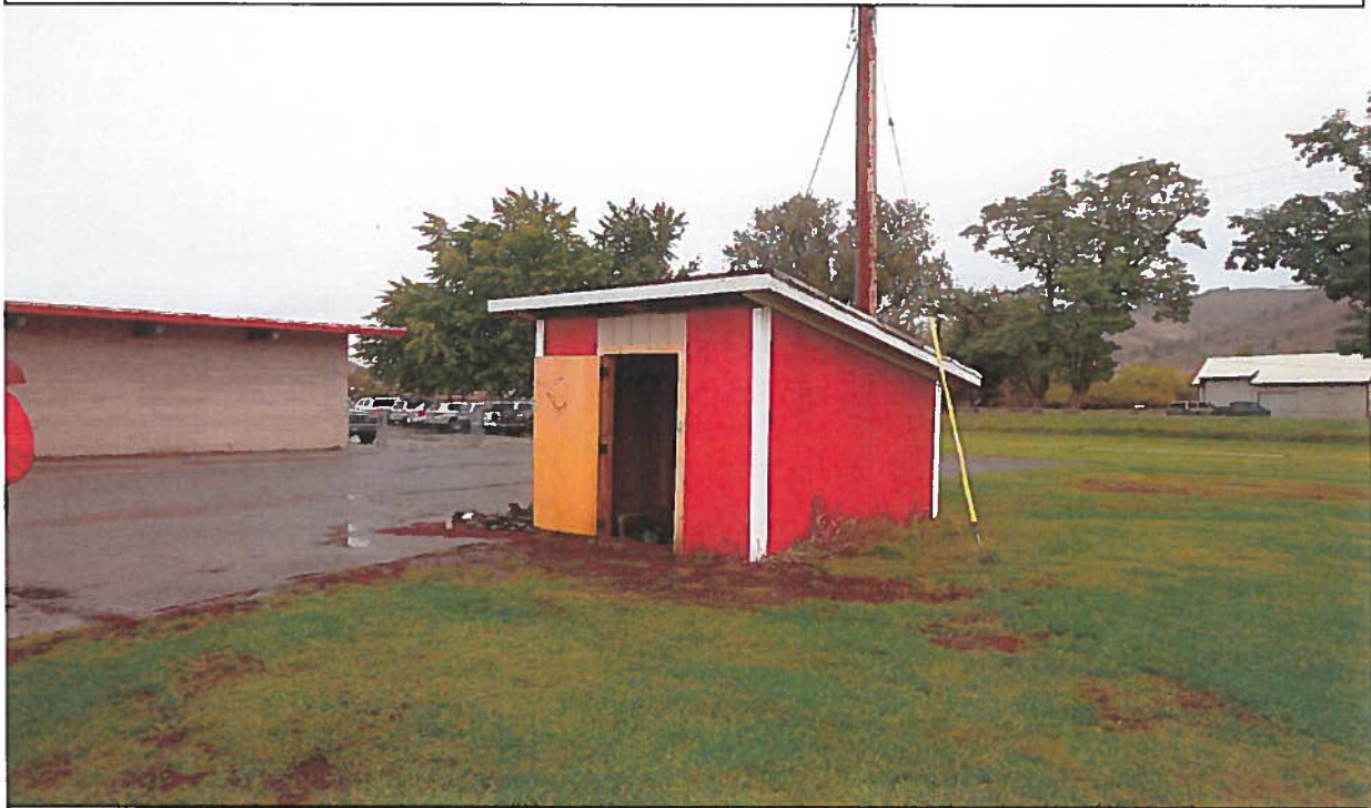
Point of Diversion: View northeasterly of the well and pump house located near the northeast corner of the football and track field.
