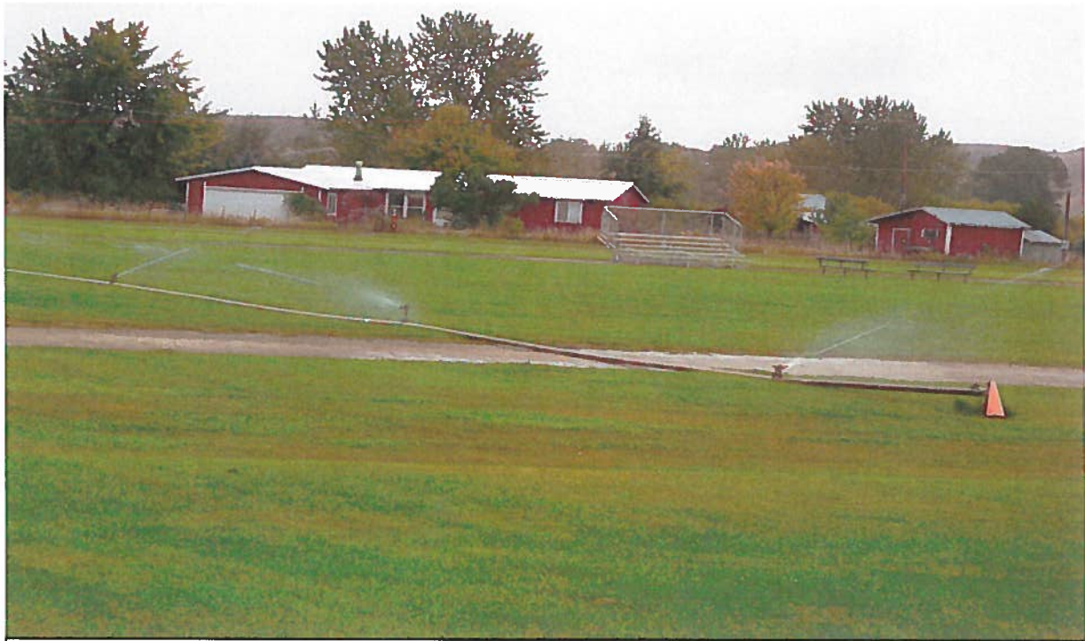
Place of Use: View southwesterly of the 3" hand line irrigation system irrigating the football and track field. The irrigation system operates with 22 Nelson sprinklers per setting.
