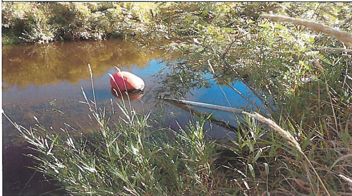
Point of Diversion: View northerly of the 4" flexible suction line in Squaw Creek. A large flotation device is attached to the 4" suction line to suspend the 4" intake off the bottom of Squaw Creek.
