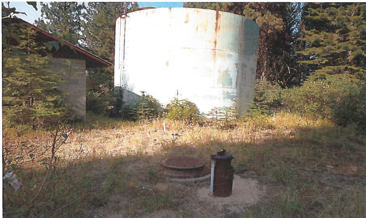
View southwesterly of a ground water well, known as the 'Main Well', a 50,560-gallon steel water storage tank, and the pump house. A concrete manhole/vault near the well contains a water storage tank bypass valve and a water system flush valve.
