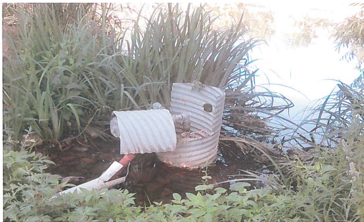
Lot owners have individual pump to irrigate from the large pond. This is one of them.
