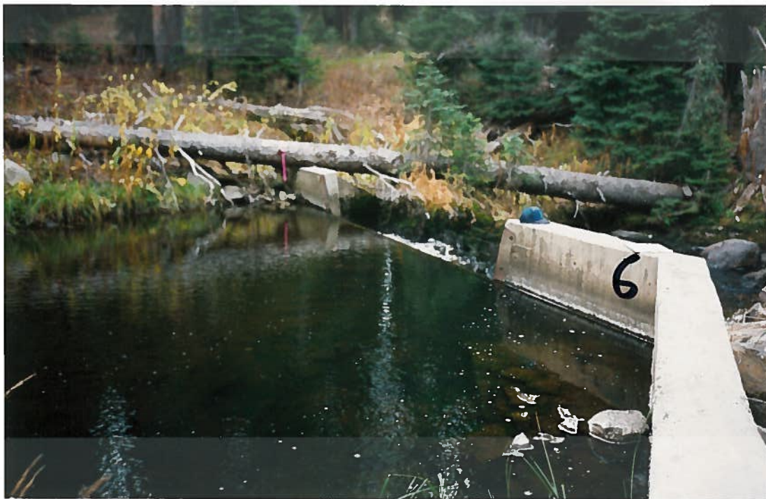
⑥ Cipolletti weir located roughly 200' to 225' downstream from dam, weir blade 12'-15' in width
