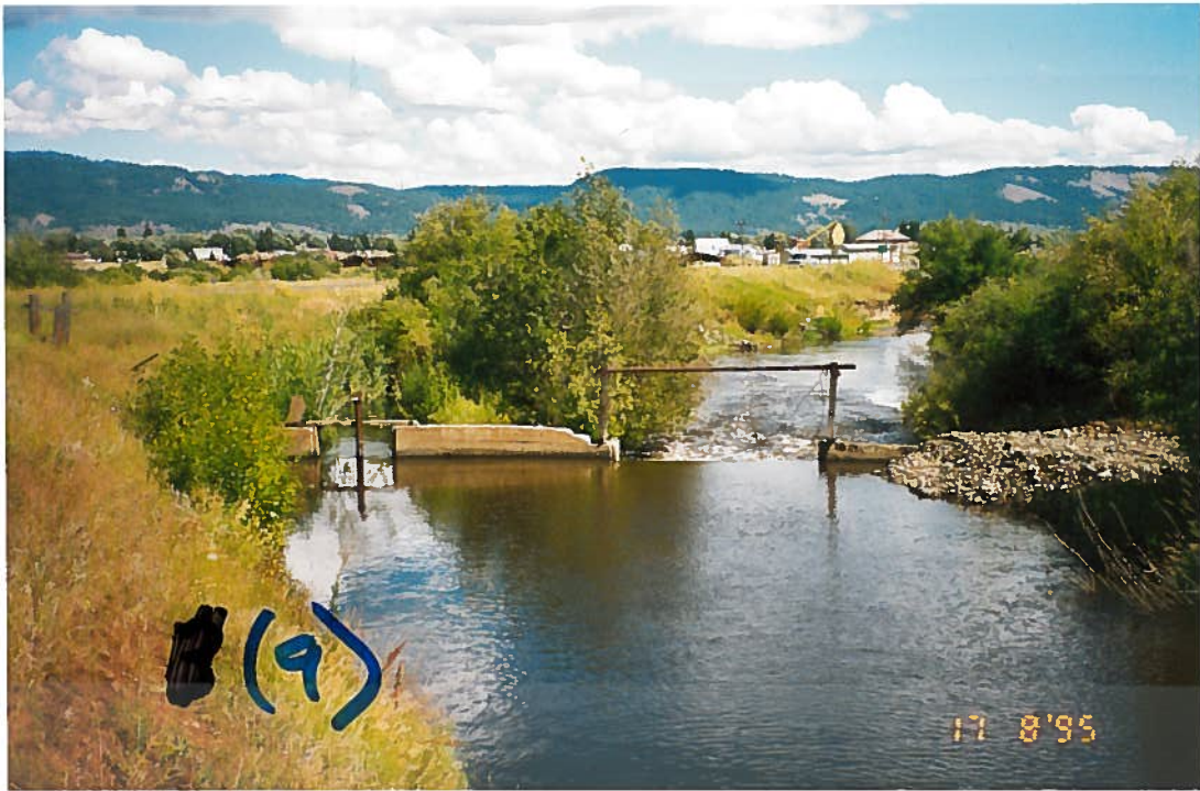
⑨ Westside Ditch headgate structure
