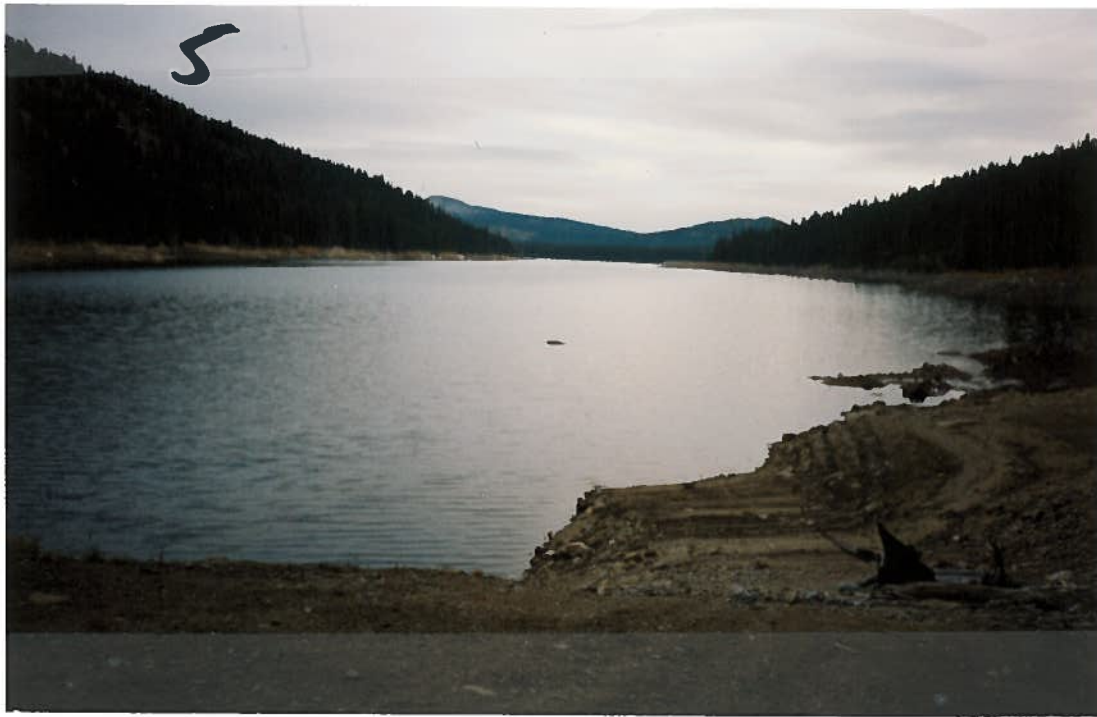
⑤ view of reservoir from SE end of dam
