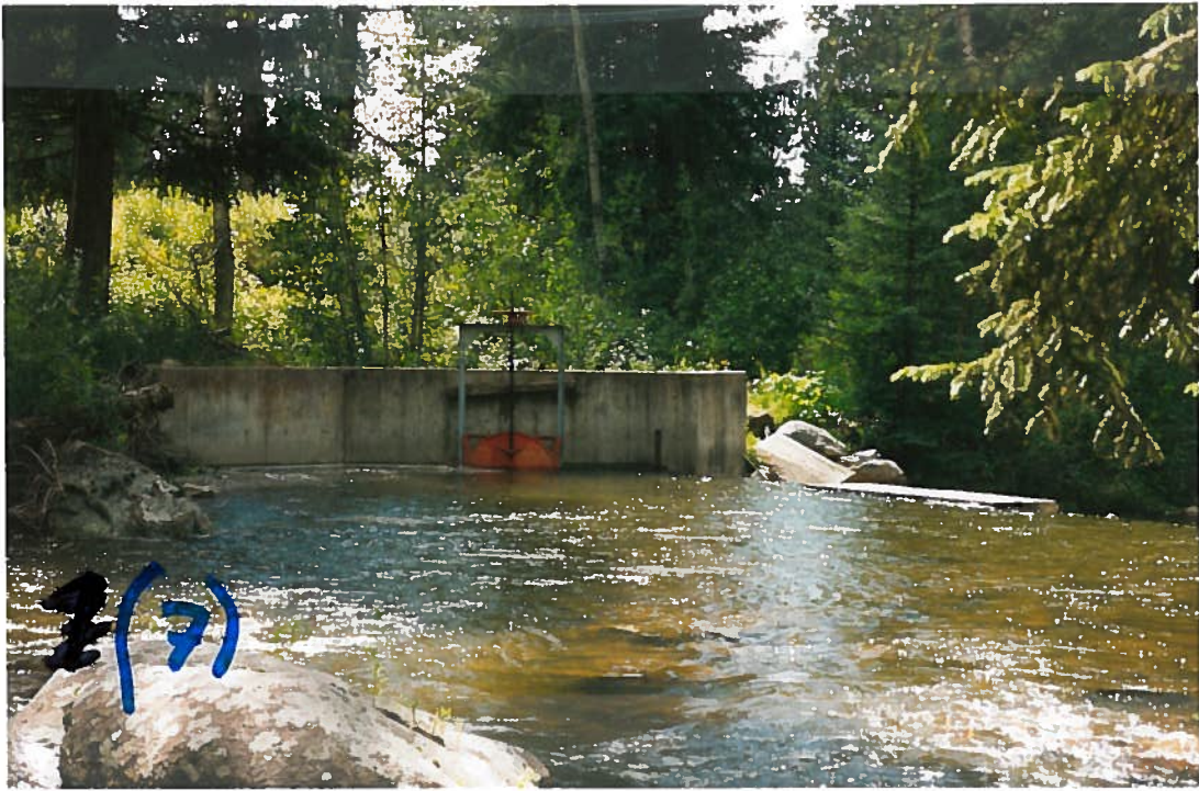
⑦ Southside Ditch headgate structure
