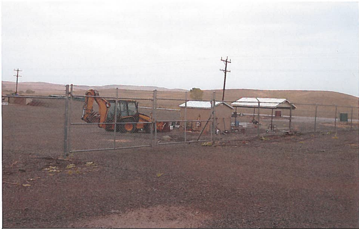
Place of Use: View southeasterly of the solid waste transfer site. Water is pumped to a frost-free hydrant near the structure fire protection.
