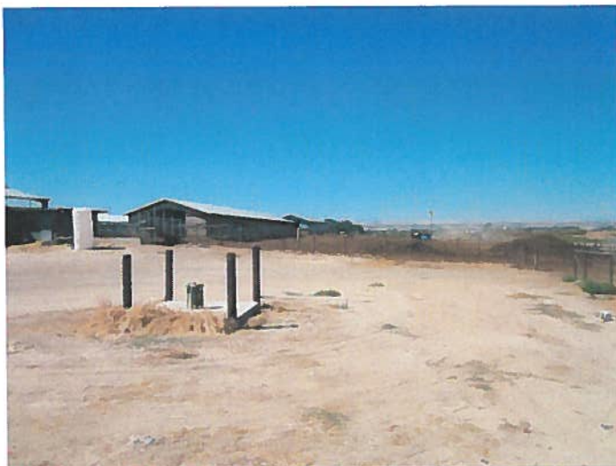
Primary well looking west
