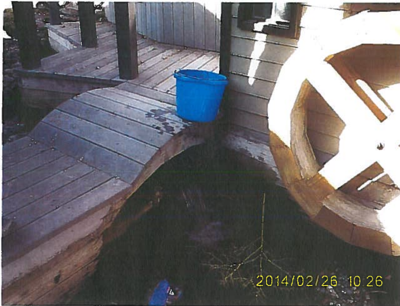
Photo 7809. Location of Bucket-and-stopwatch flow measurement. A small rock was placed after taking the photograph, to deflect the stream to be narrow enough for bucket capture.
