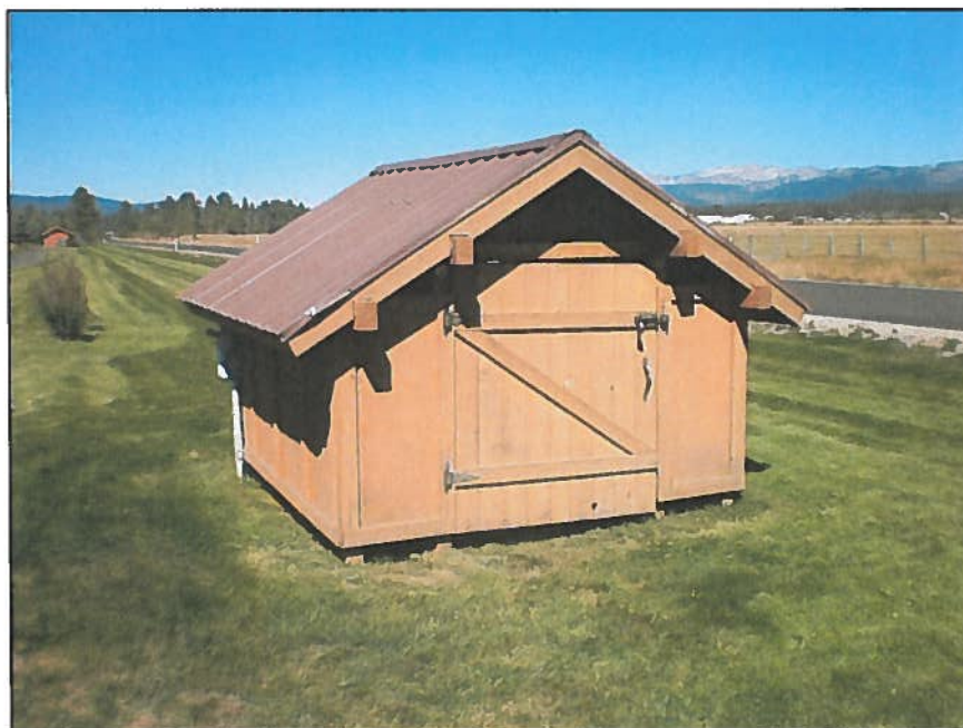
Figure 10: Secondary irrigation pump house.
