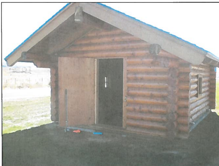
Figure 6: Irrigation well house.
