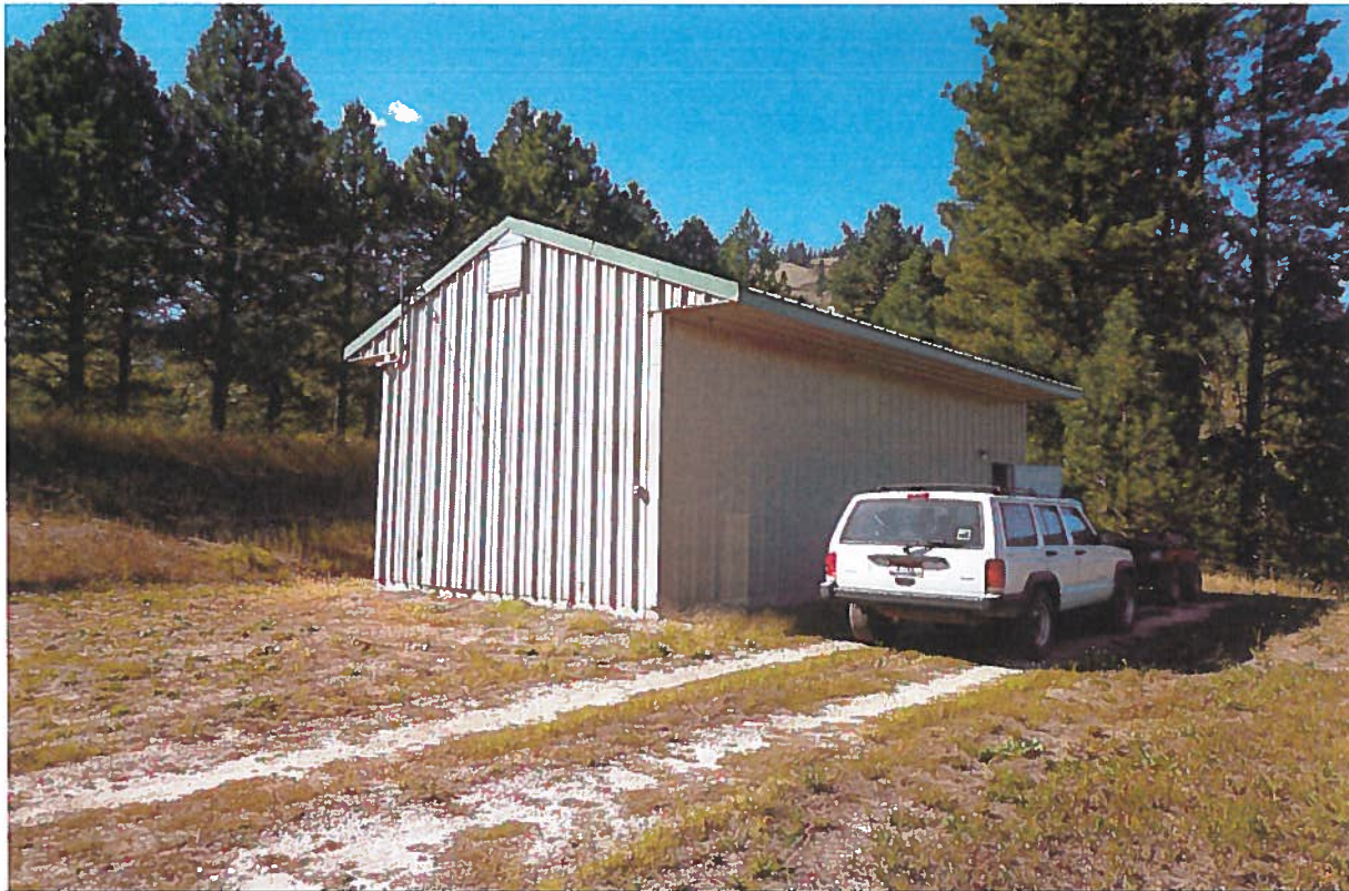
View northwesterly of the water treatment and water system control building. The water treatment facilities include a slow sand filter tank and a clarifier tank for chlorination.
