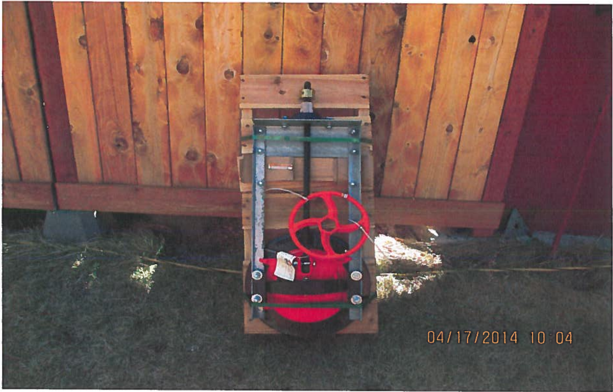
Replacement sluice gate for return flow pipe.
