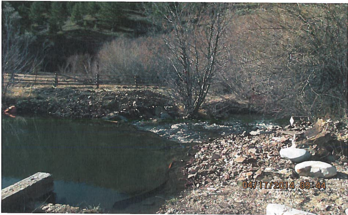
Close up of the Diversion Dam
