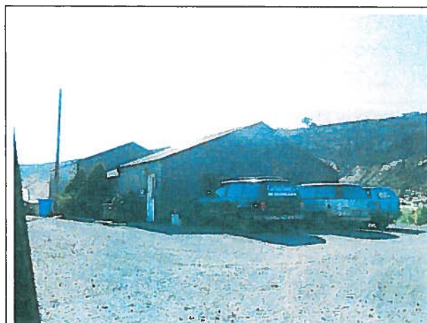
October 21, 2008 Office & old parts area
