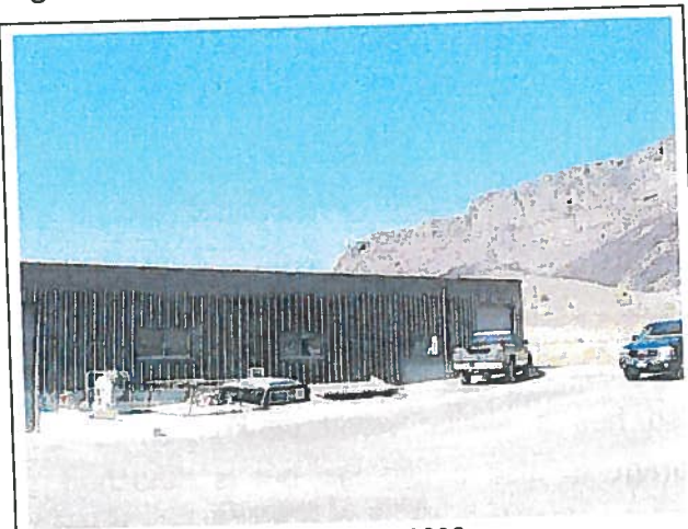
October 17, 2008 Hatchery building
