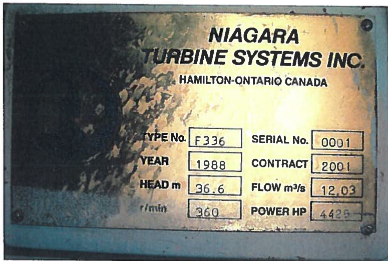
Magic Reservoir Hydroelectric Turbines 1, 2, and 3
