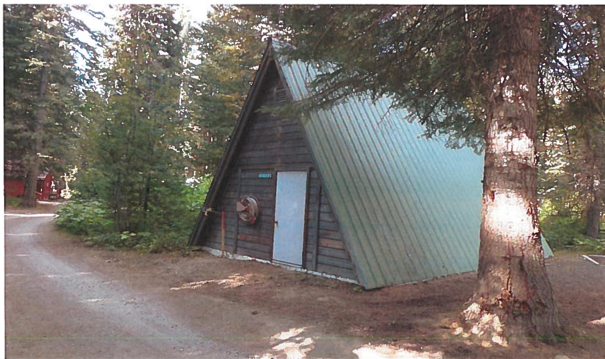
View southwesterly of the pump house. The ground water well is located approximately 100' westerly of the pump house.
