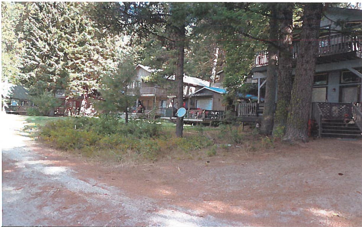
Place of Use: View northwesterly of a few of the 19 homes served by the ground water well.
