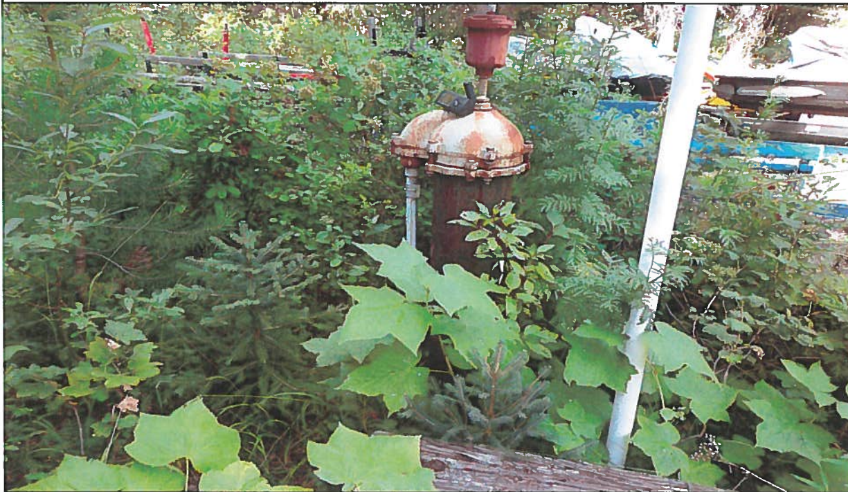
Point of Diversion: View southerly of the ground water well which provides water for domestic use for 19 homes.
