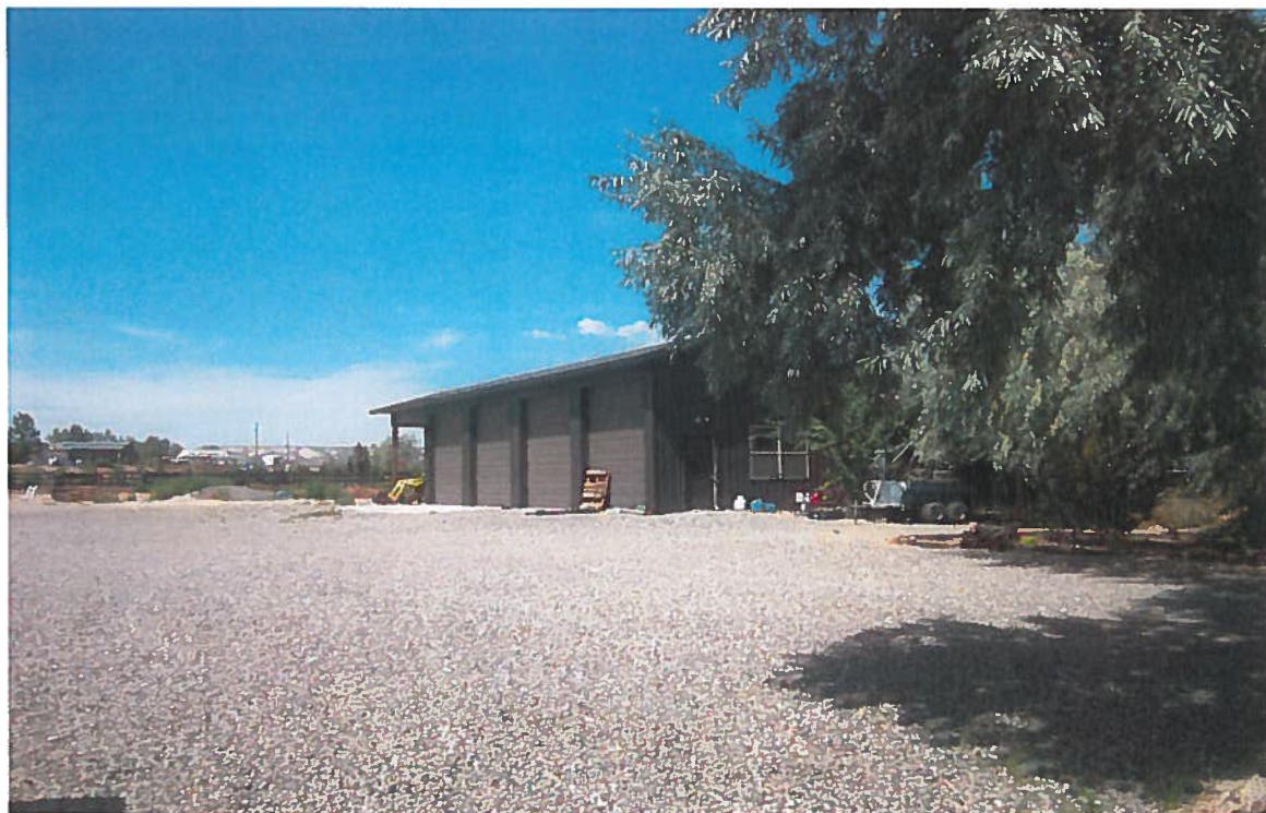
The shop is heated by the hot water. After heating the home, the water is piped to the shop , seen here. There is also an underground drain that runs from the shop to the fish pond.
