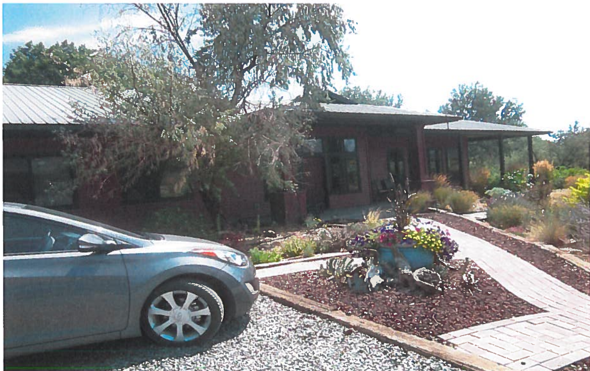
Hot water is used to heat the house, shown here.
