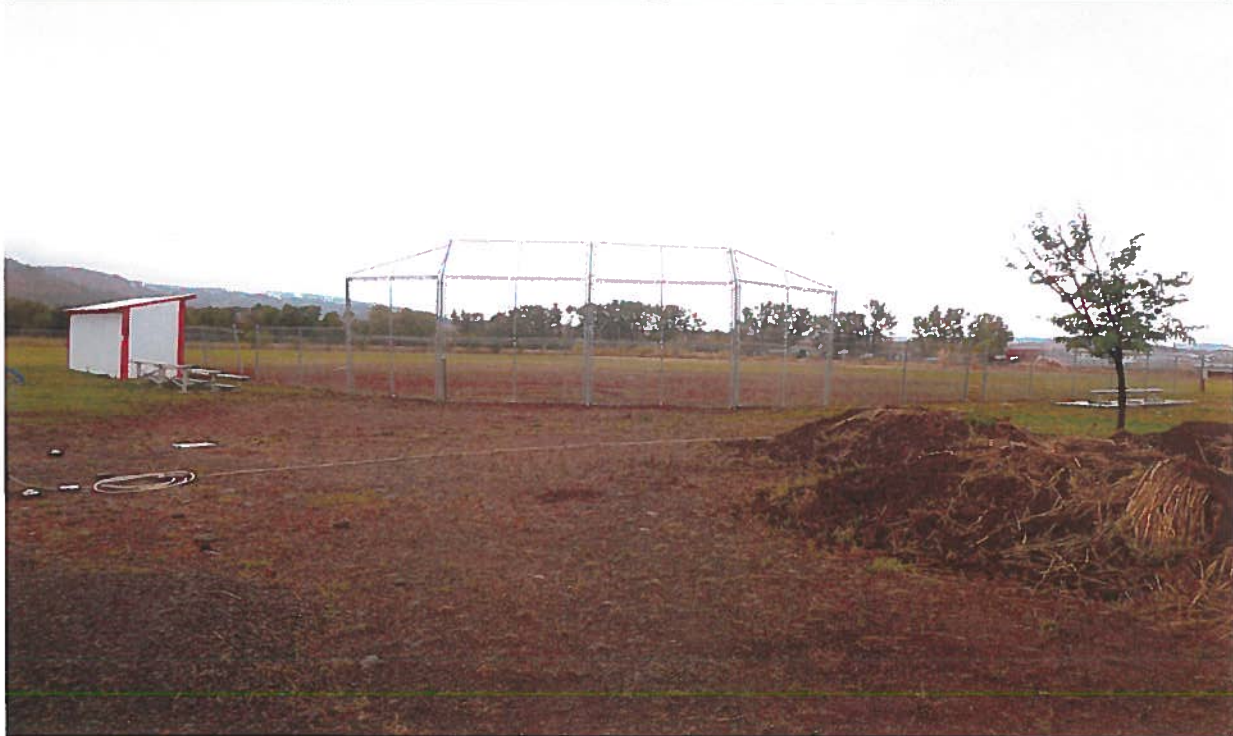
Place of Use: View northwesterly of the northerly baseball field irrigated from the ground water well. The pressurized irrigation system is comprised of Rainbird Falcon rotor sprinklers.
