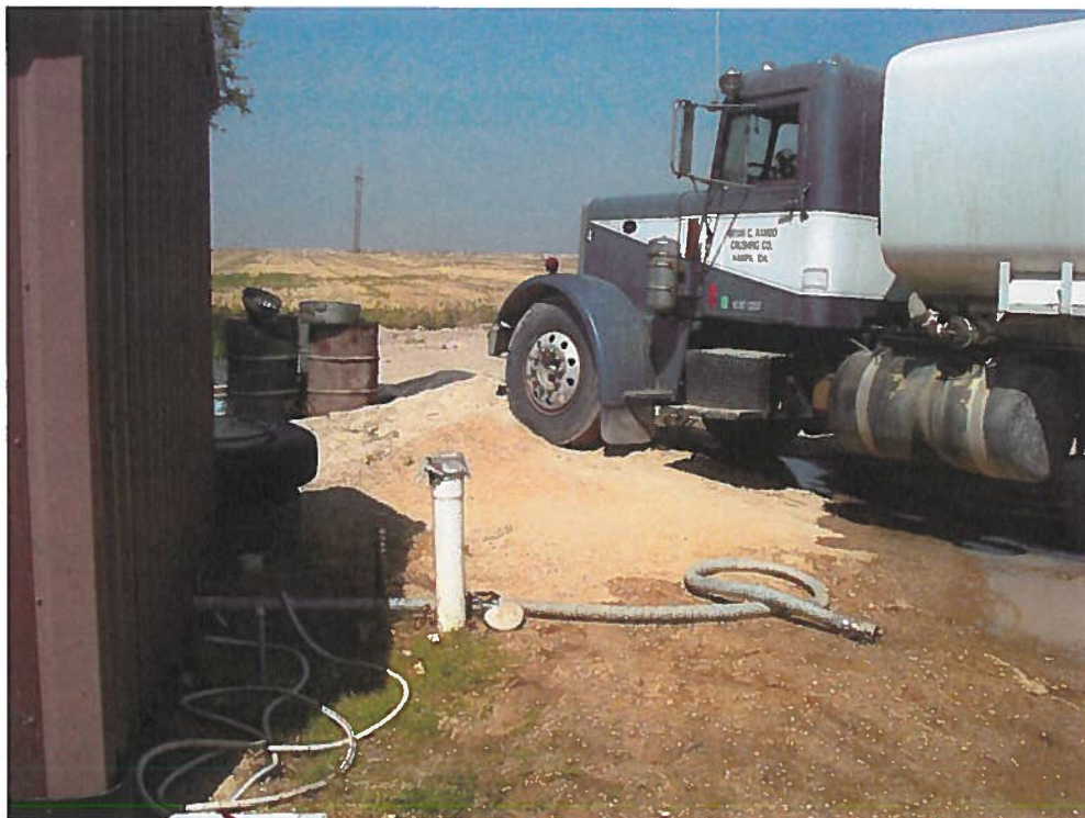
63-11764 Exam 8/27/2012: Hose east side of pump house used to fill tanker trucks to take water to gravel operation.
