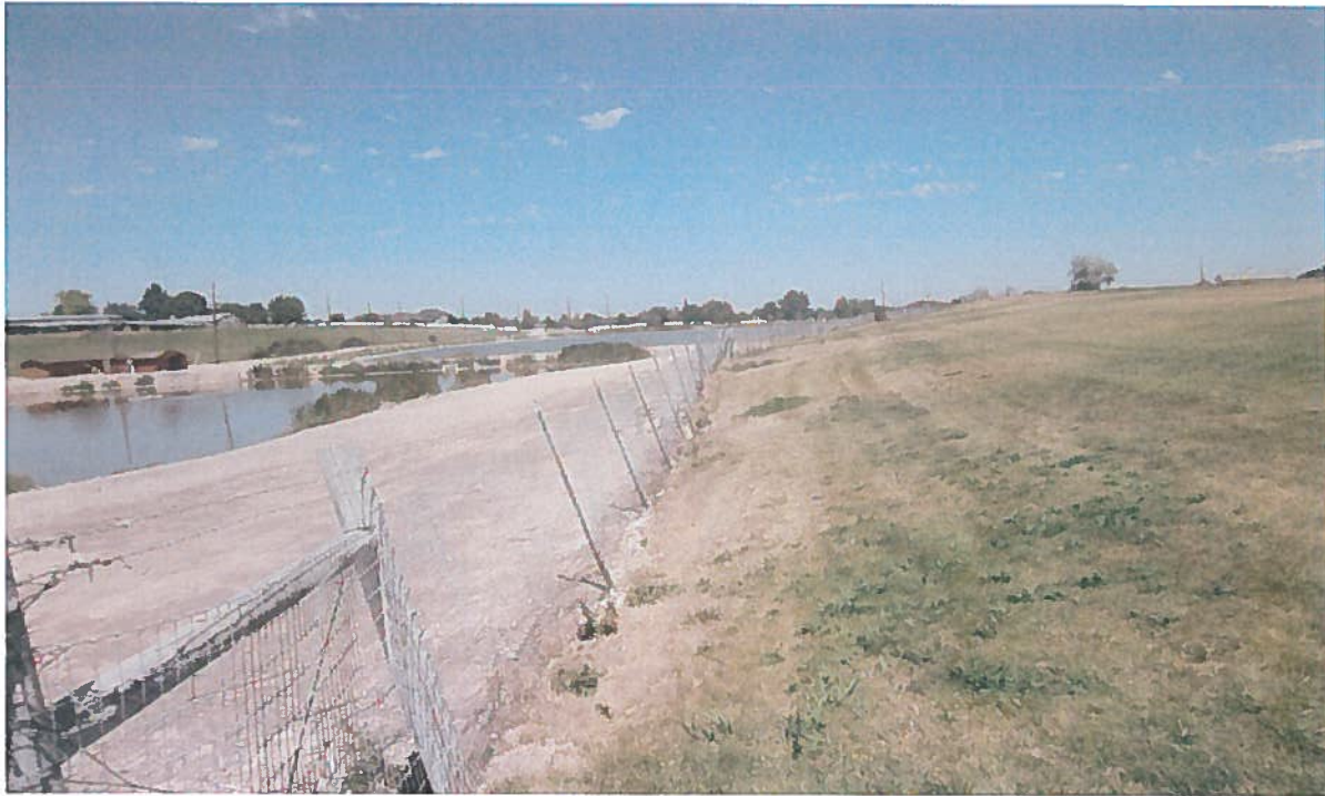
Looking north – south pond is a treatment pond. Water is diverted from the north pond for irrigation. Pump house seen middle left of photo.
