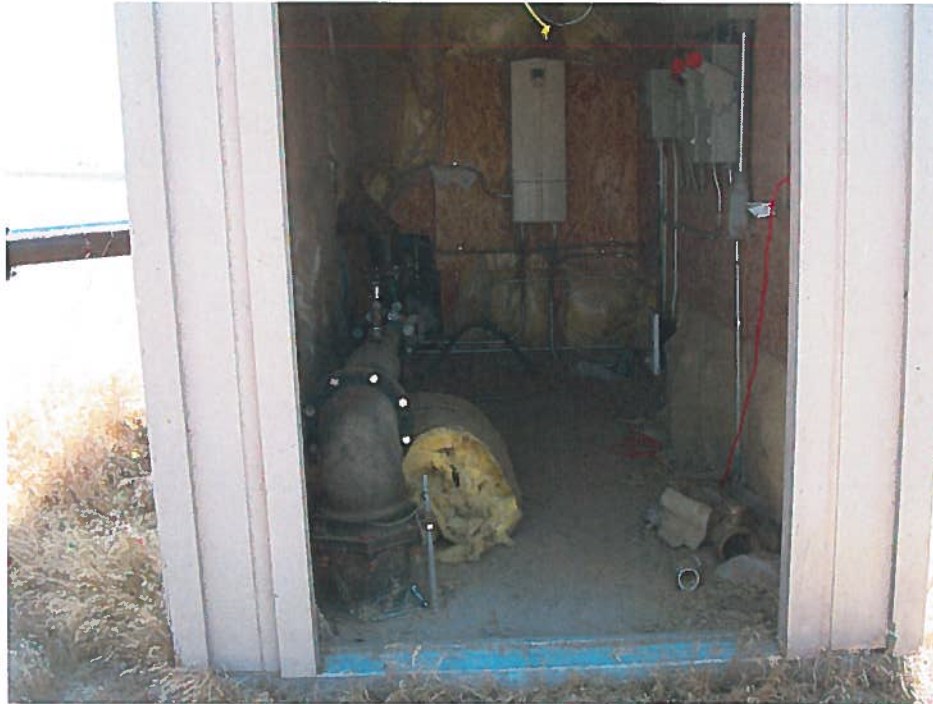
63-31982 Exam 8/30/2012: POD pump house facing south. POD well at back end (south) portion of pump house, casing not visible at surface.
