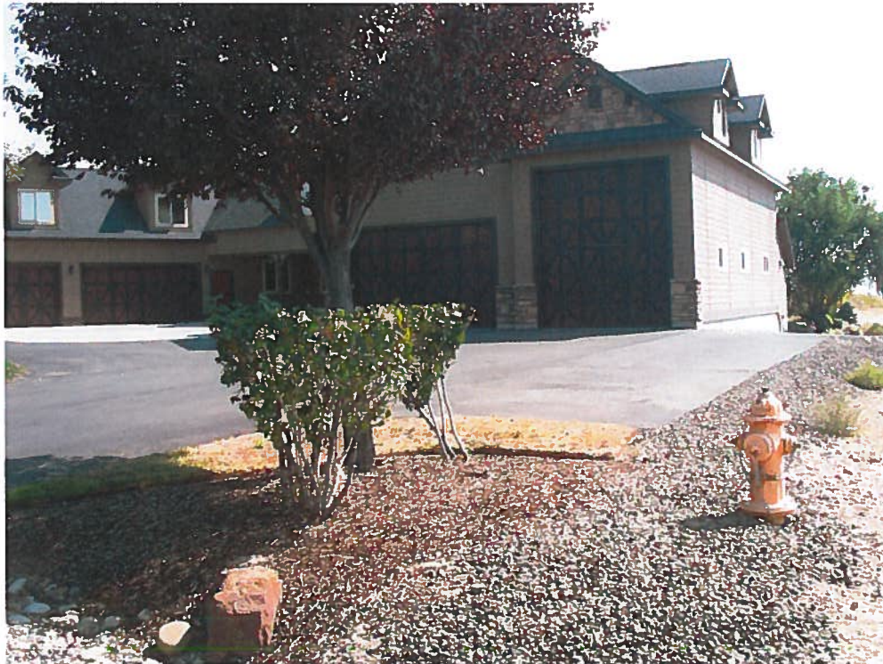
63-31982 Exam 8/30/2012: Final fire hydrant off buried 8 inch mainline facing southeast.
