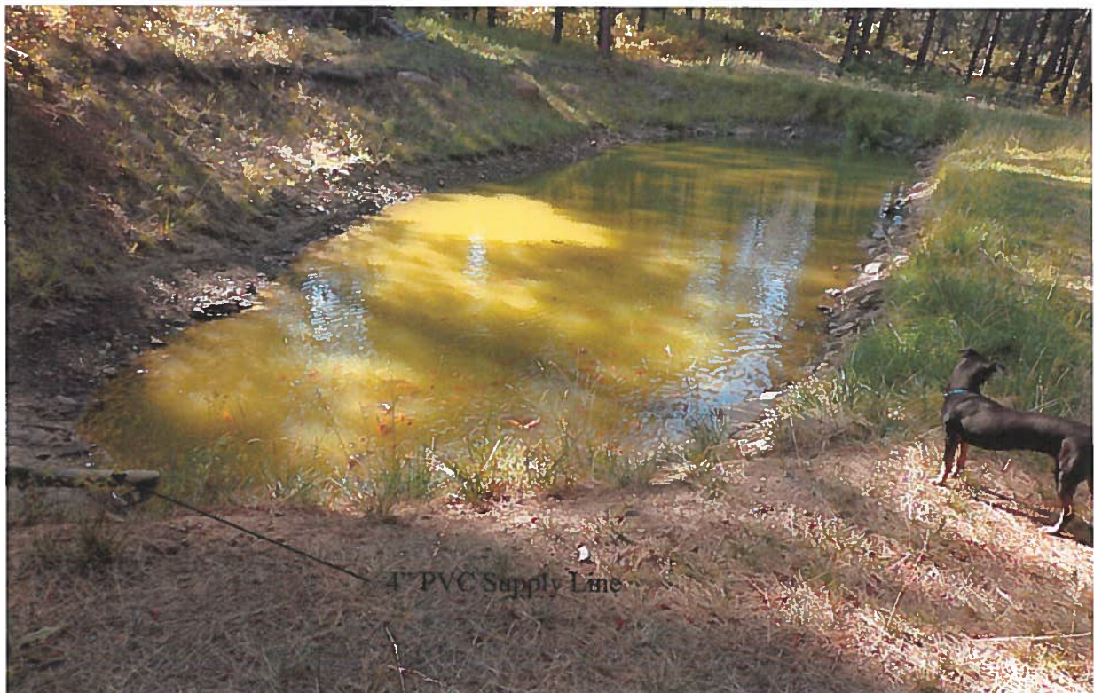
Place of Use: View of the domestic storage pond. The 4" PVC supply line is shown entering the pond. Water is discharged from the storage pond through 4" PVC pipe to 4" PVC discharge manifold located at the toe of the dam.
