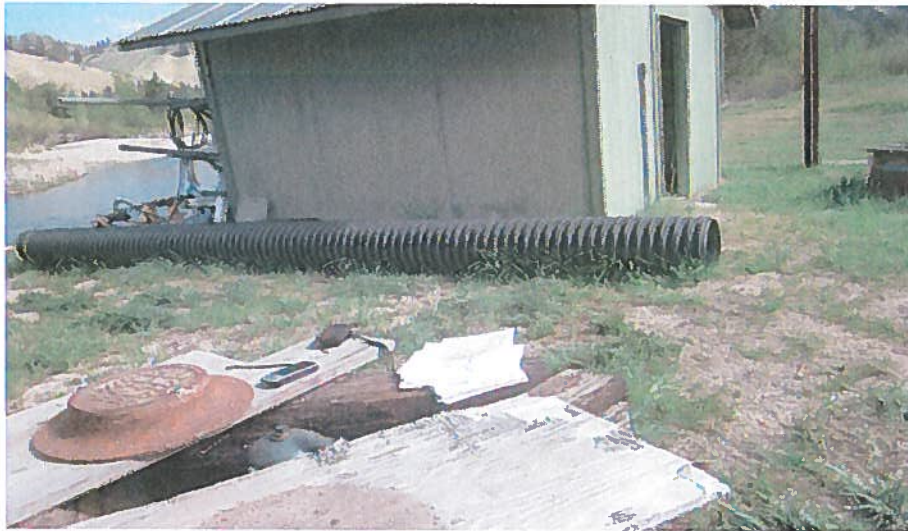
The cold water pump house and cold water well # 2, south of the pump house.
