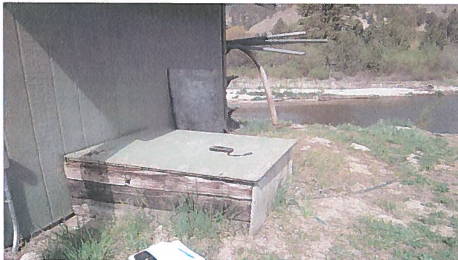
Cold water well # 1, on north side of cold water pump house.
