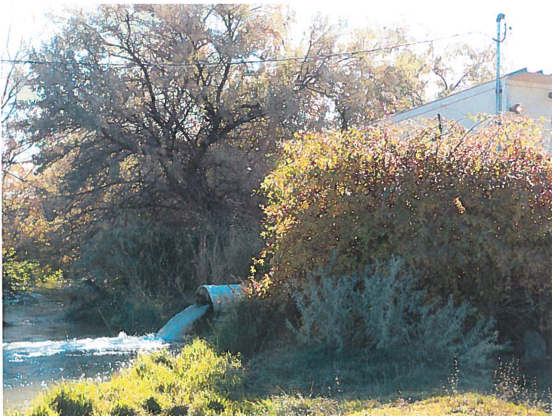
Outlet from powerhouse into Mud Creek
