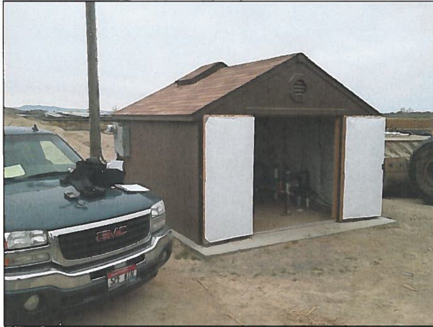
Figure 1: Well #4 is located in a pump house at T1S R1W Section 7 NESW.
