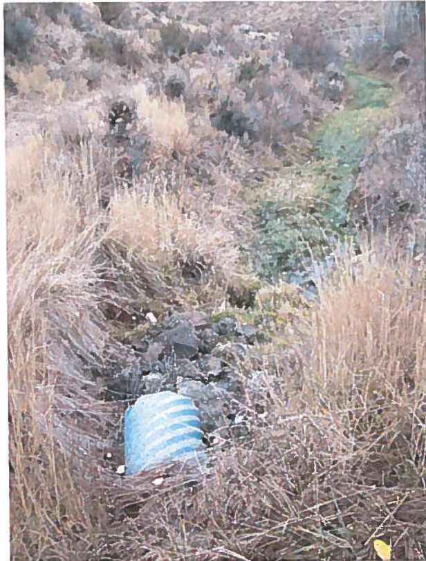
Figure 3: Downstream view of the outlet (15" CMP) and Unnamed Stream Channel
