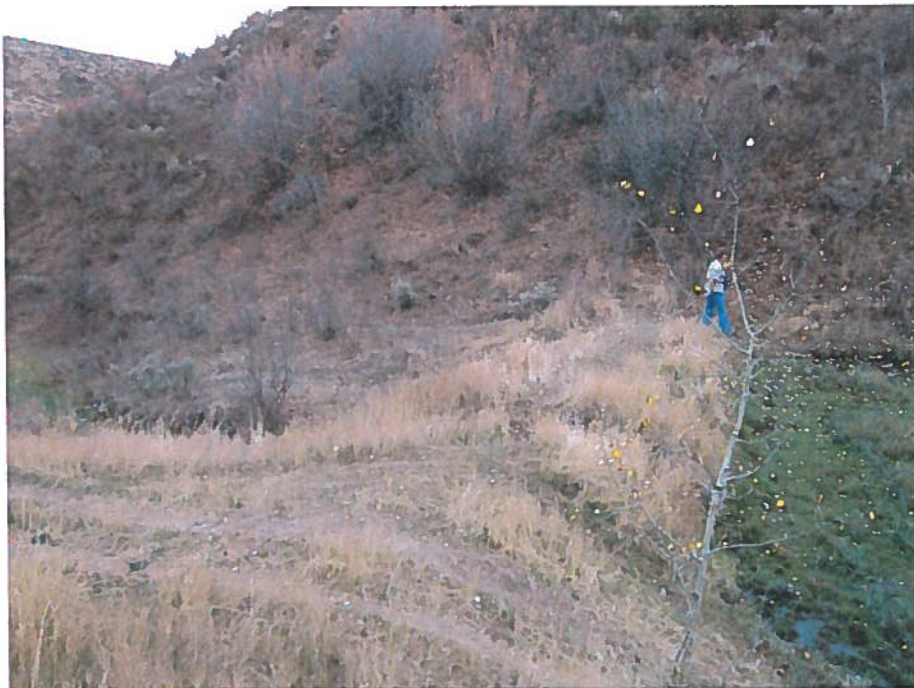
Figure 2: view of the Embankment (POD) across the Unnamed Stream Tributary to Van Camp Creek
