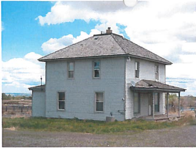
Main house at dairy
