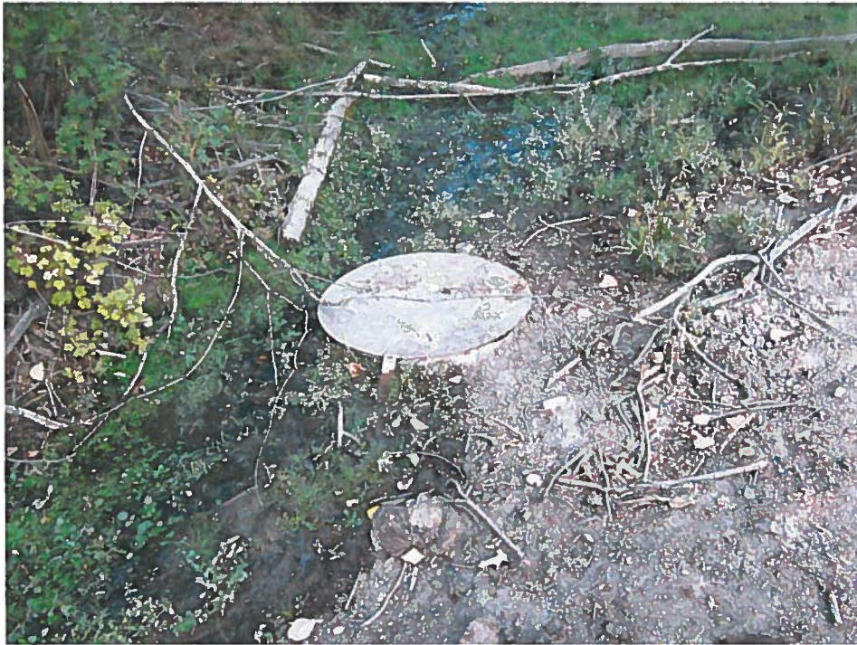
Figure 1. Point of Diversion (Culvert/Headbox) in Spring Gulch Creek Channel
