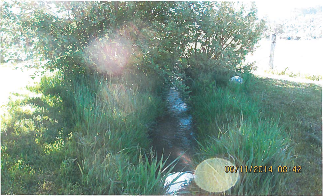
Pond Inlet Pipe, looking East
