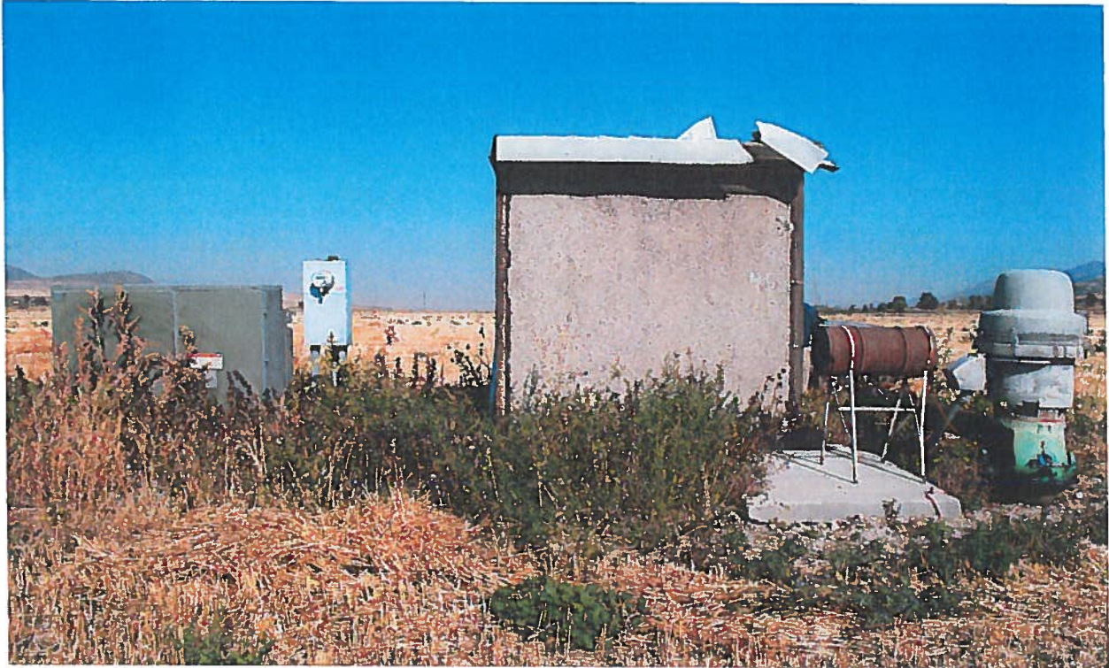
Back Side of well and Pump house
