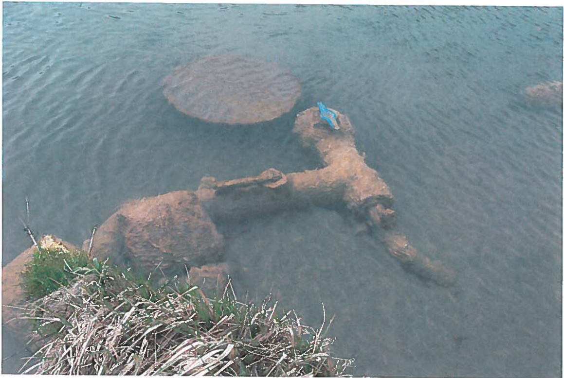
outflow end of 6-in pipe
