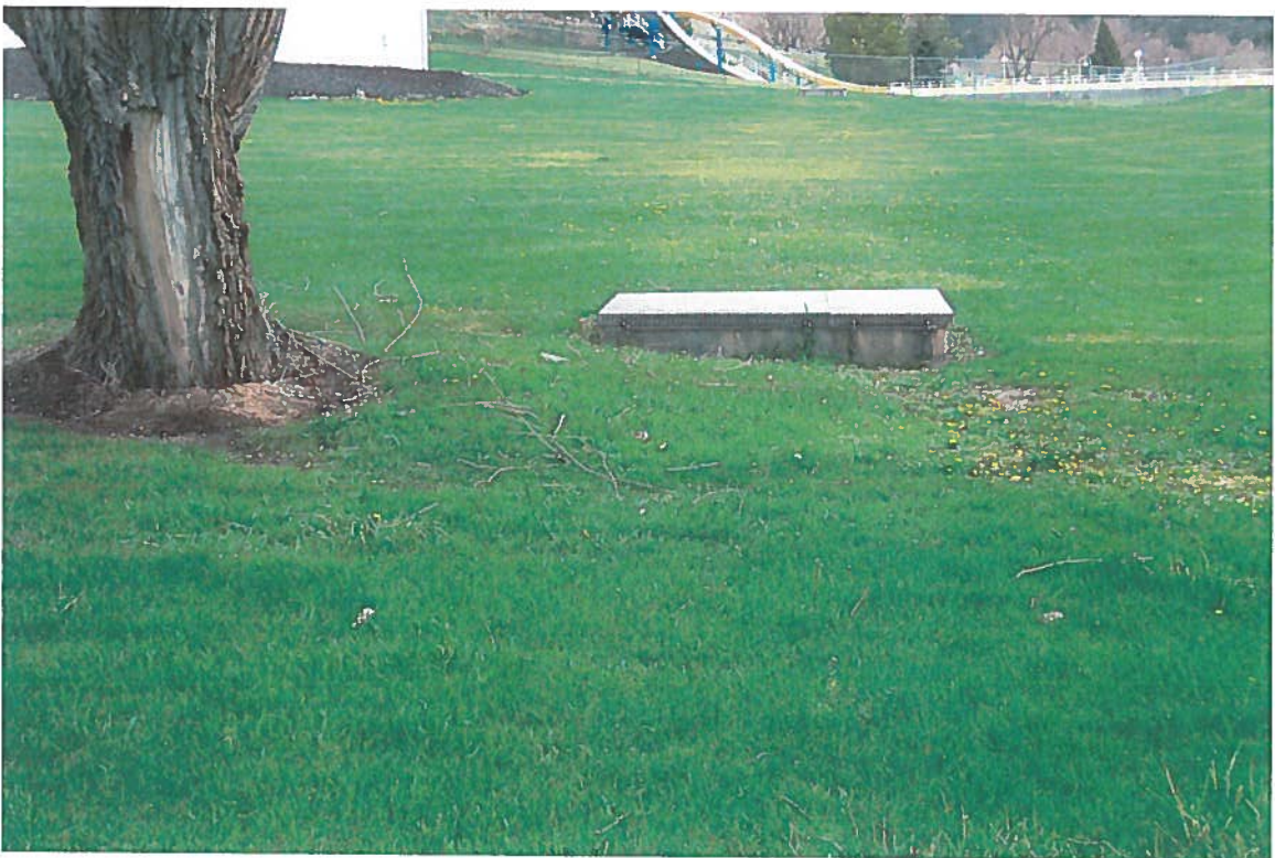
Valve box - point of diversion
