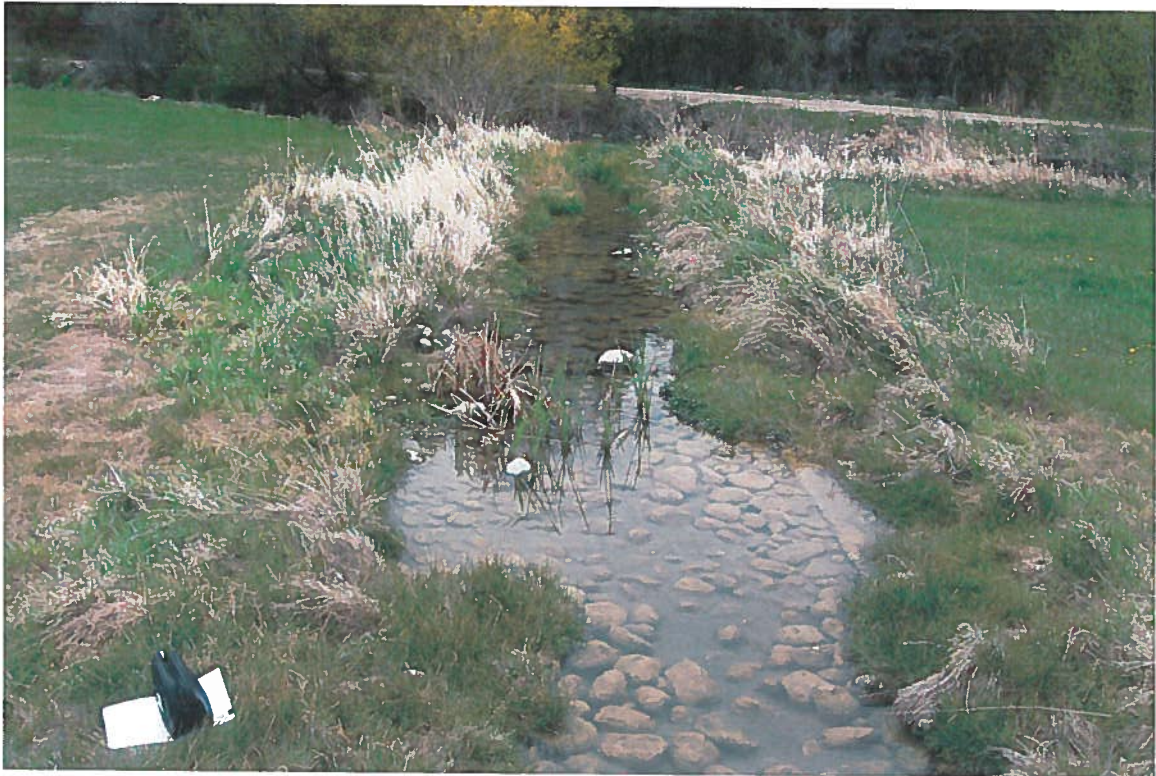
ditch from pond to Portneuf River
