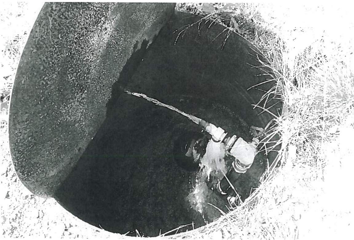
Clear cr. Spring PL Pressure tap, Valve
