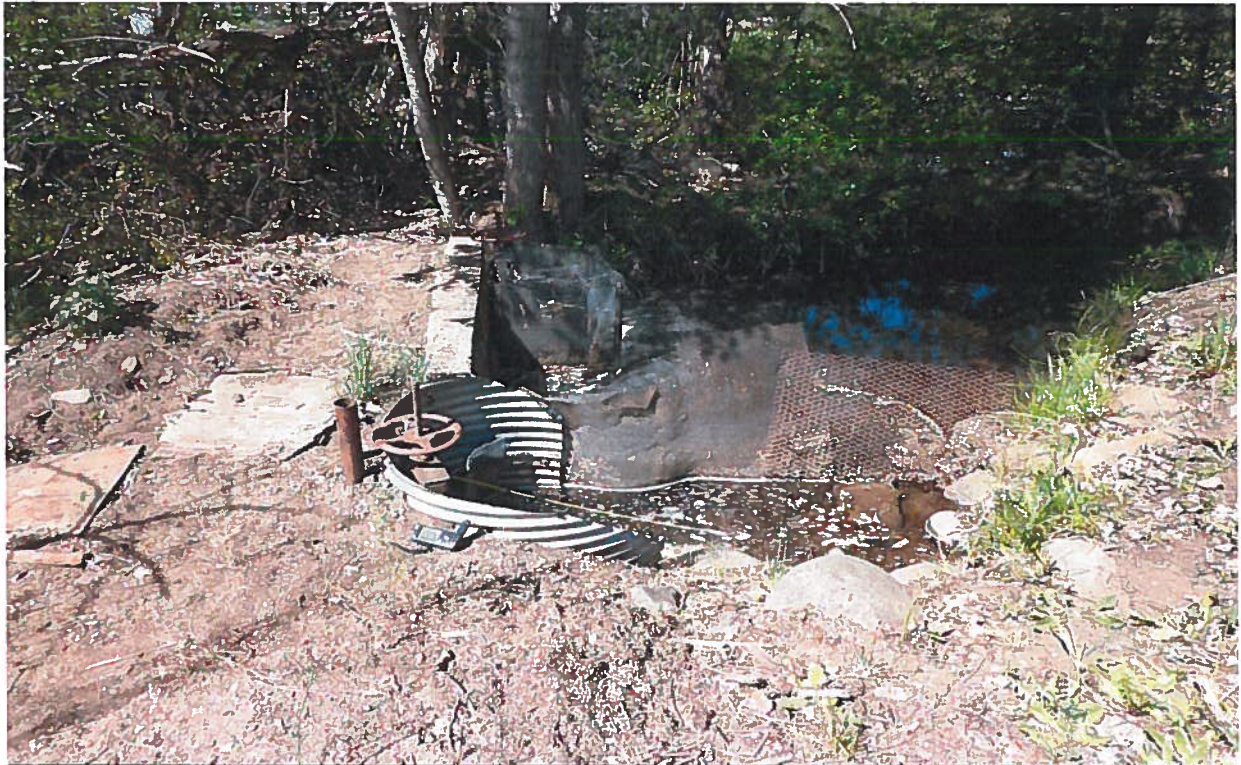
Point of Diversion: View westerly of the concrete diversion structure located at the end of the discharge channel from Rush Creek. The right holder's head gate is located in the half-section of 42" CMP. A short section of 10" PVC extends from the channel to the 42" CMP.
