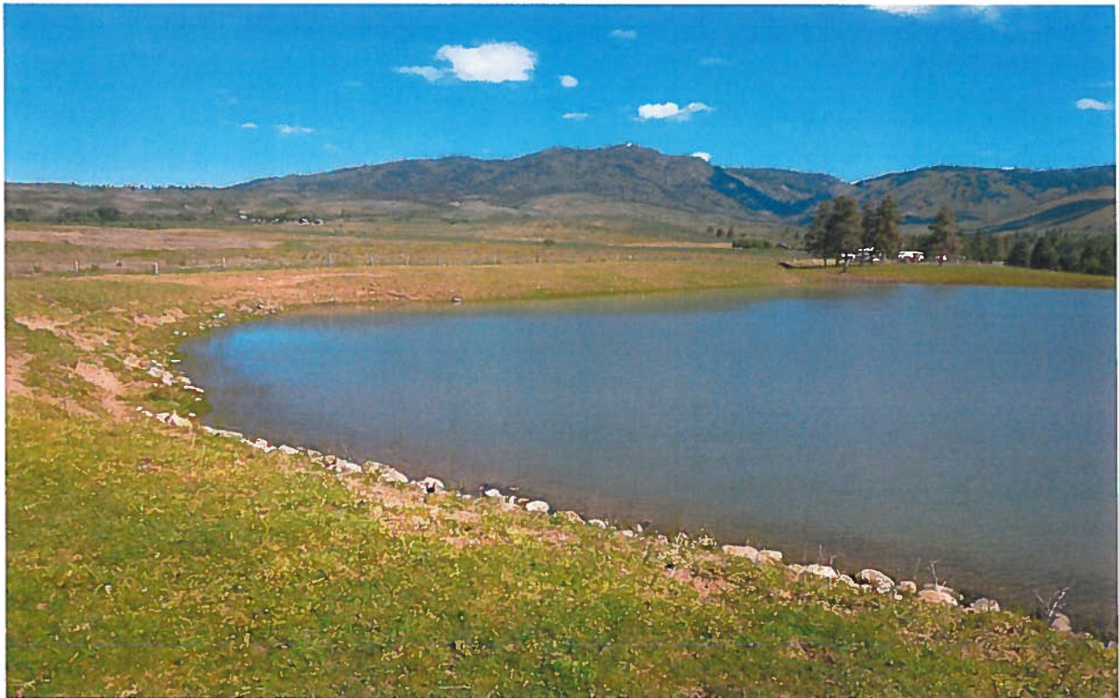
View southeasterly of the irrigation storage pond. The maximum pond depth is 25'.
