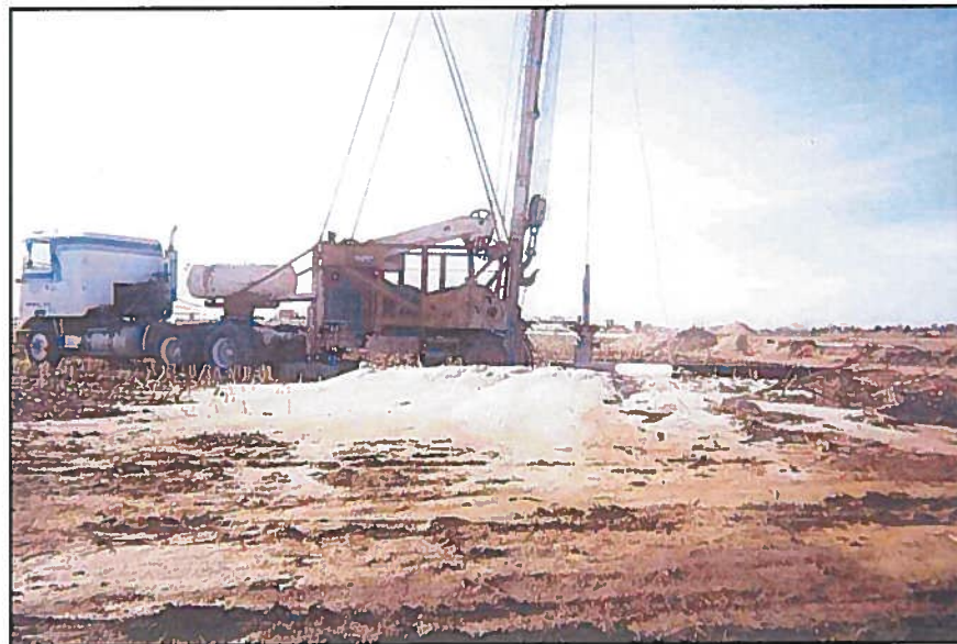
February, 2002 photograph of the cable-tool drill-cuttings pile for the Sundance irrigation well. This well was completed to similar depths as the City's Well #23.
