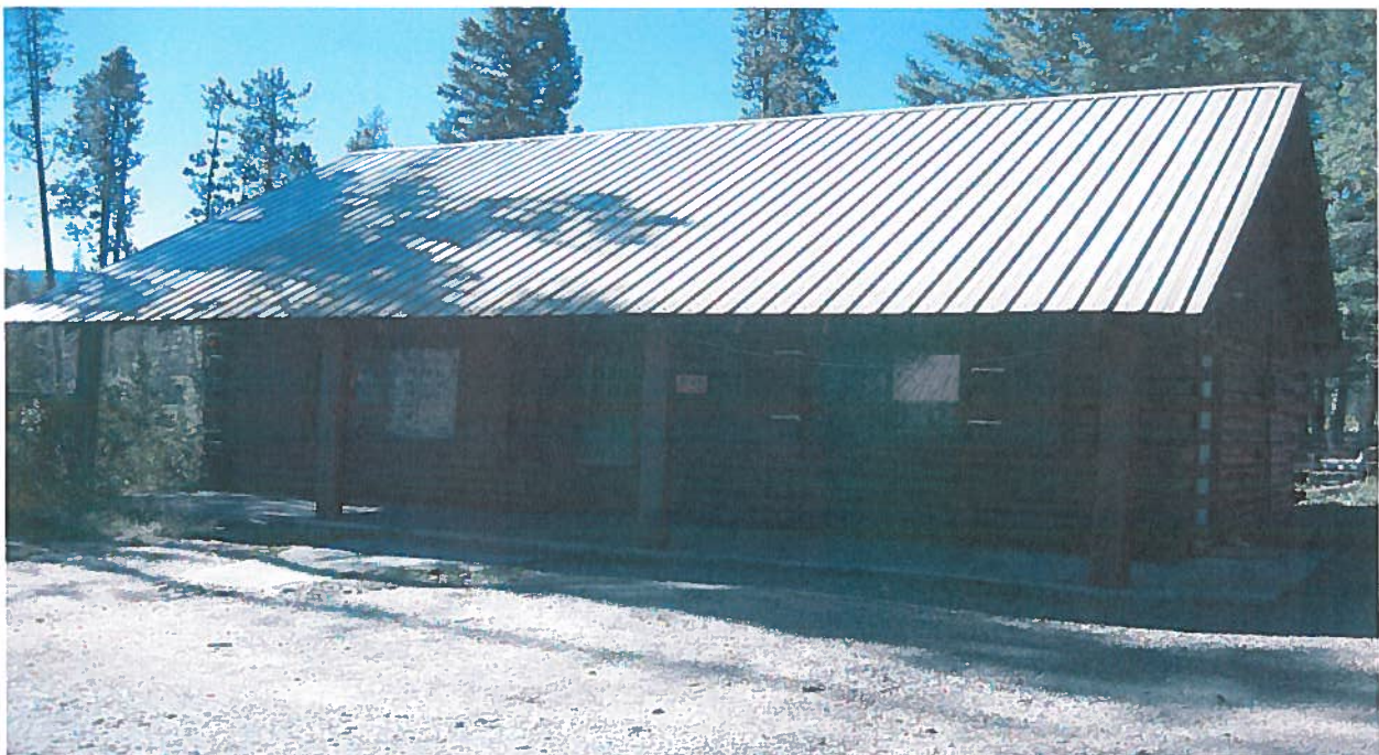
Below: Caretaker's Cabin
