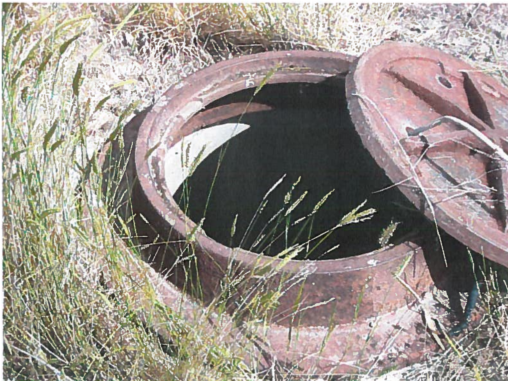
Well Pit with Manhole Cover Removed
