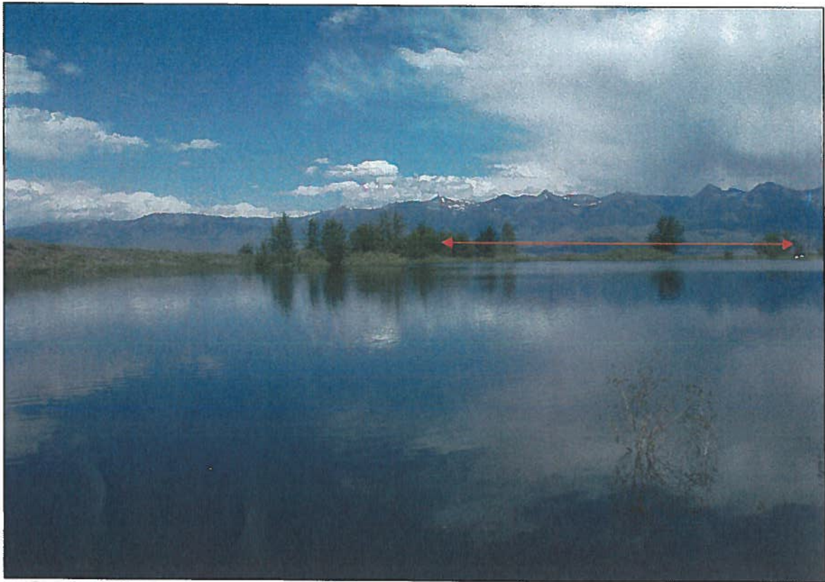
Photo 6 (6/25/09) - View from the back of the reservoir looking east, toward the crest of the embankment. Note the elevated water level referenced by the submerged vegetation.
