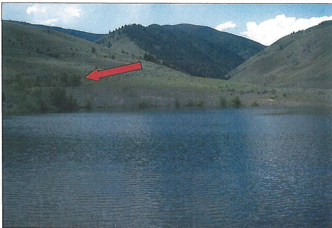
Photo 2 (6/25/09) - Upstream view from dam crest looking across the reservoir to the primary source of water, supplied by a developed, artesian spring (shown by arrow).
