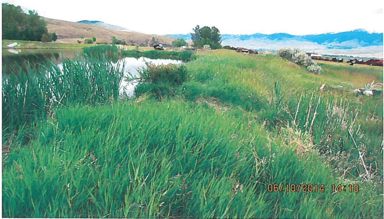
Dam, looking North
