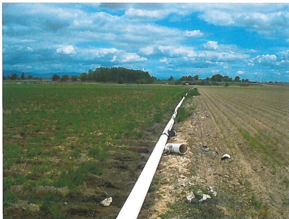
63-11707 Exam 5/23/2012: Portion of POU facing east.
