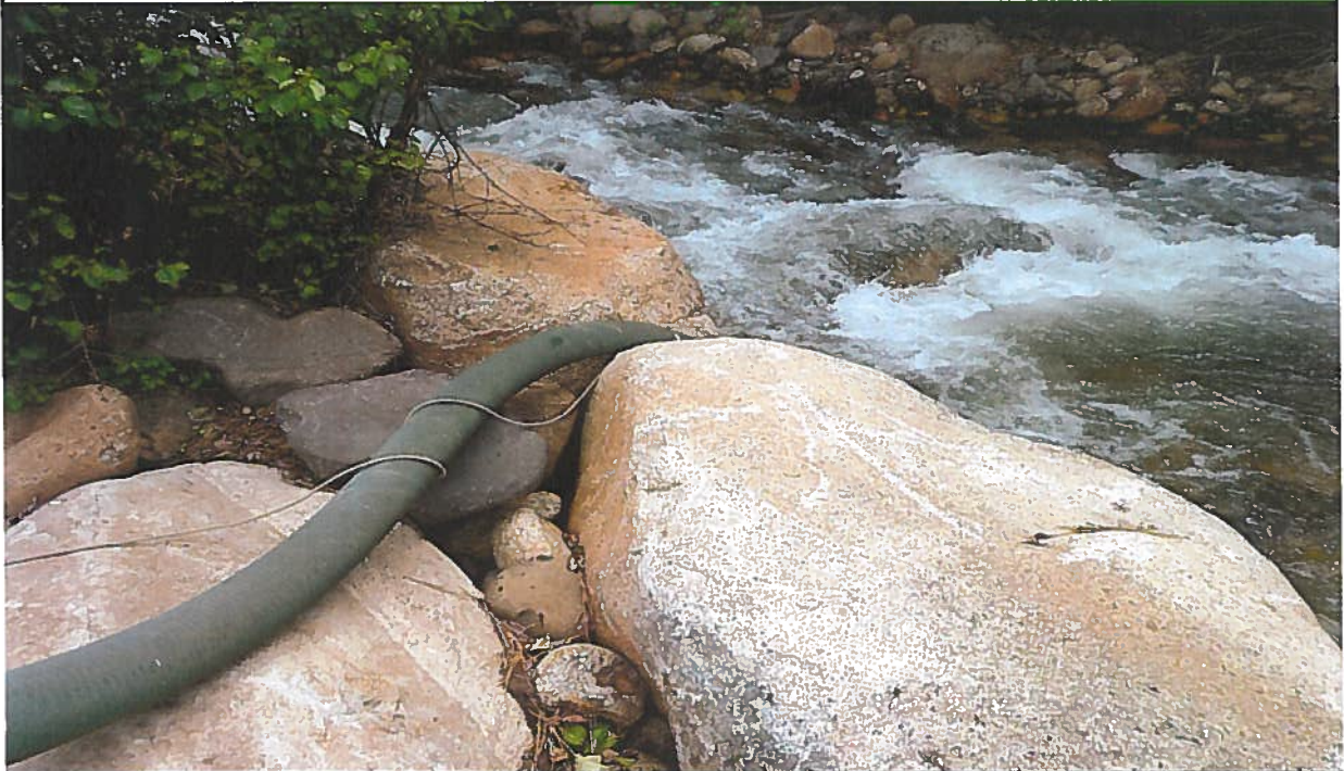
Point of Diversion: View southerly of the 4" flexible hose suction line in East Pine Creek.
