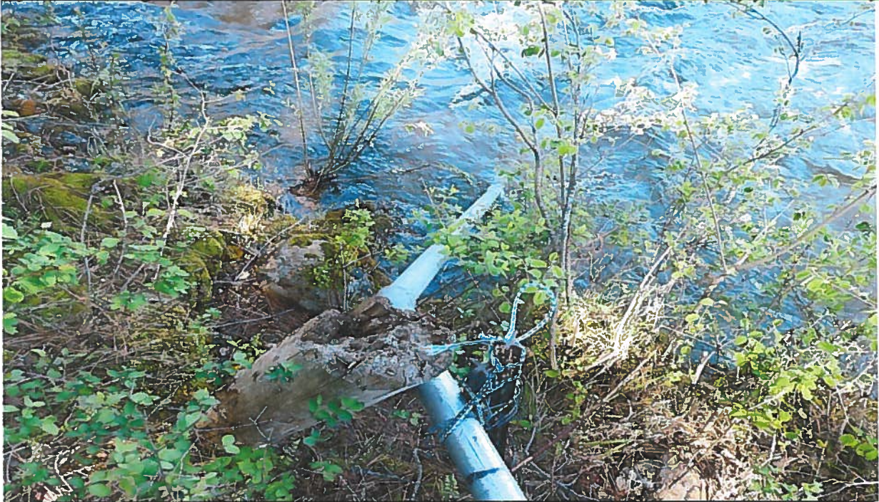
Point of Diversion: View northwesterly of the 2" steel suction line in the Middle Fork of the Payette River.
