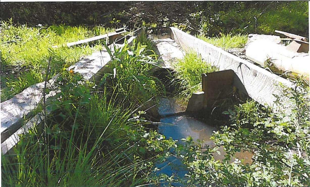
View southerly of the Cipolletti weir and water diverted from Timber Creek discharging through the 4' section of 12" concrete pipe. A section of 8" PVC pipe conveys water from the pool downstream of the weir to an irrigation storage pond.
