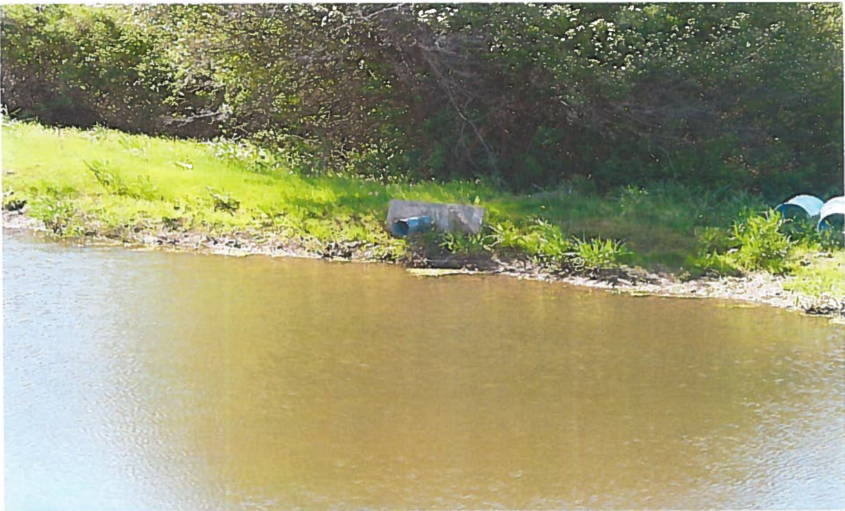
View southeasterly of the 8" CMP overflow pipe located on a dike between the storage pond and Timber Creek.
