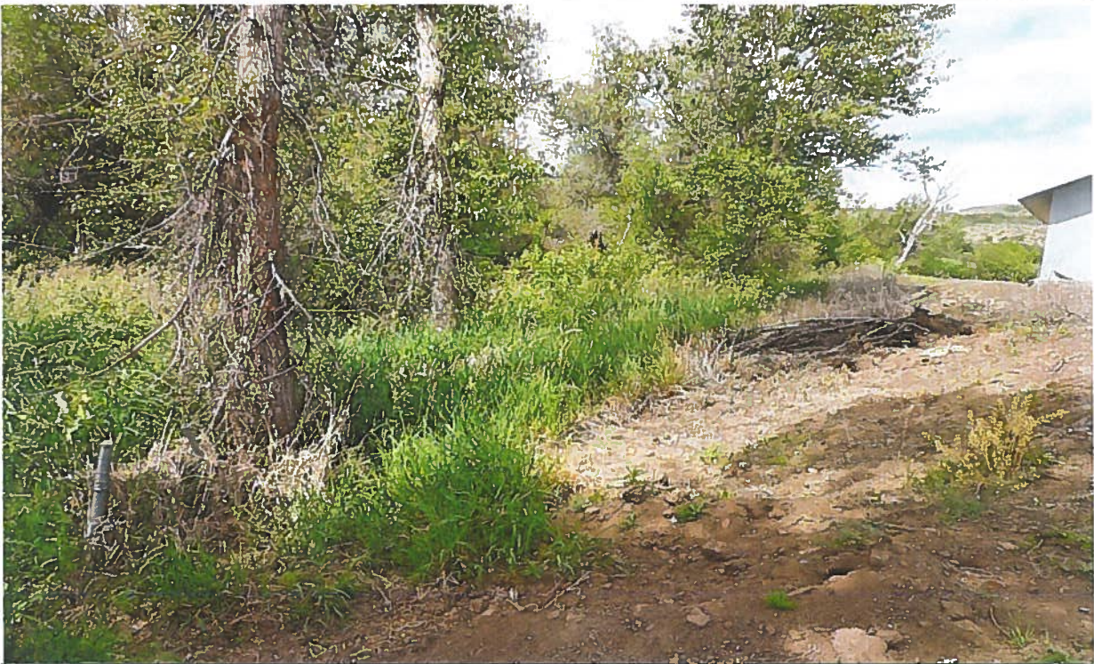
View westerly from the pumping station of the drainage area which discharges water to an 8" perforated pipe. The water is conveyed by the 8" perforated pipe to the concrete manhole sump. The building to the right is the chlorination treatment building.
